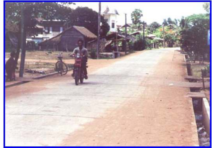
Image 3 – Bamboo Reinforced Concrete Paving
