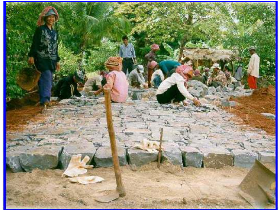
Image 2 – Dressed Stone Paving under Construction
