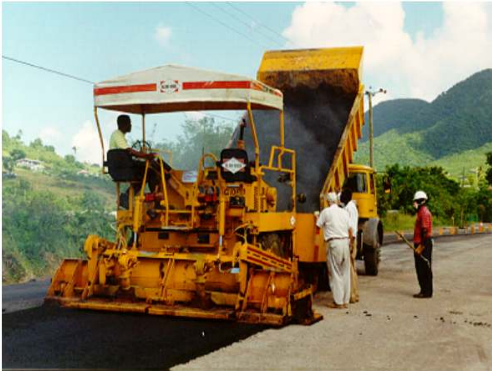
Photo 6. Truck Containing Asphalt backing up to Paver.
