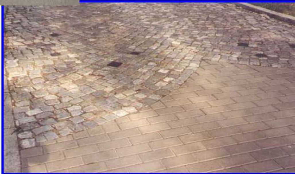
Image 5 – Pavé (small stone paving) and Concrete Block Paving
