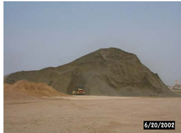
Figure 6.3 – An excessively high stockpile
