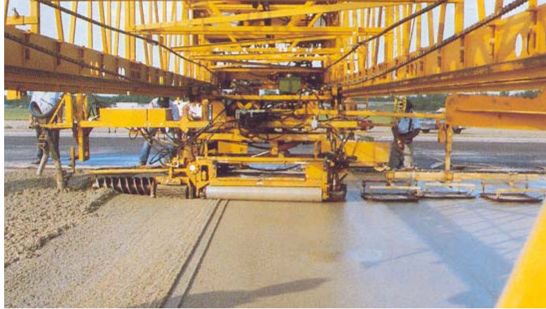
Figure 8.1 – Typical bridge deck paving operation
