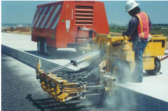
Figure 8.4 – Dowel bar installation along a longitudinal construction joint
