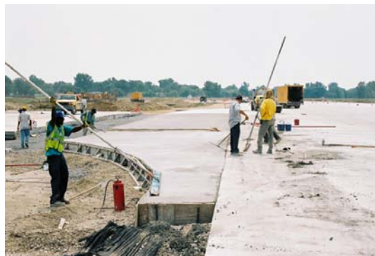
Figure 8.2 – A typical fillet construction operation
