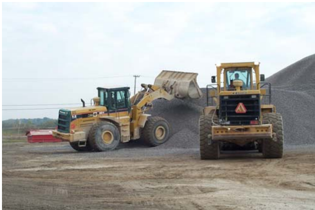
Figure 6.2 – Working the aggregate stockpile
