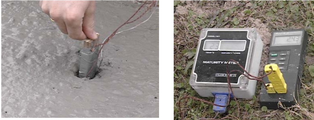
Figure 9.5 – Maturity meter testing
