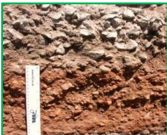
GCS base over natural gravel sub-base
