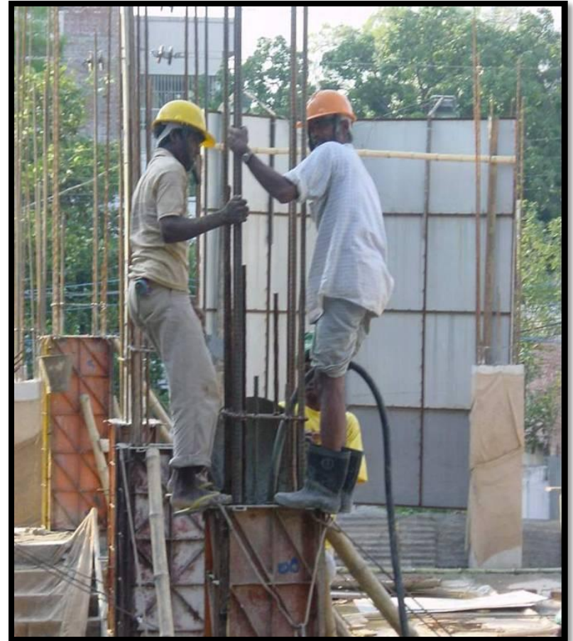
Use Of Vibrator
