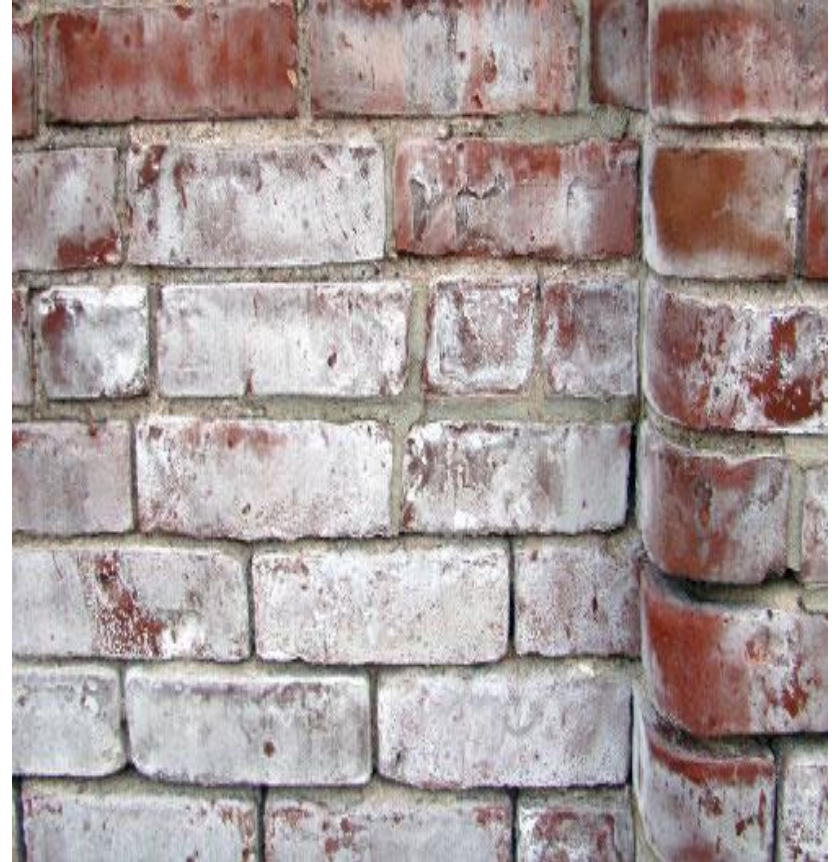
Efflorescence
