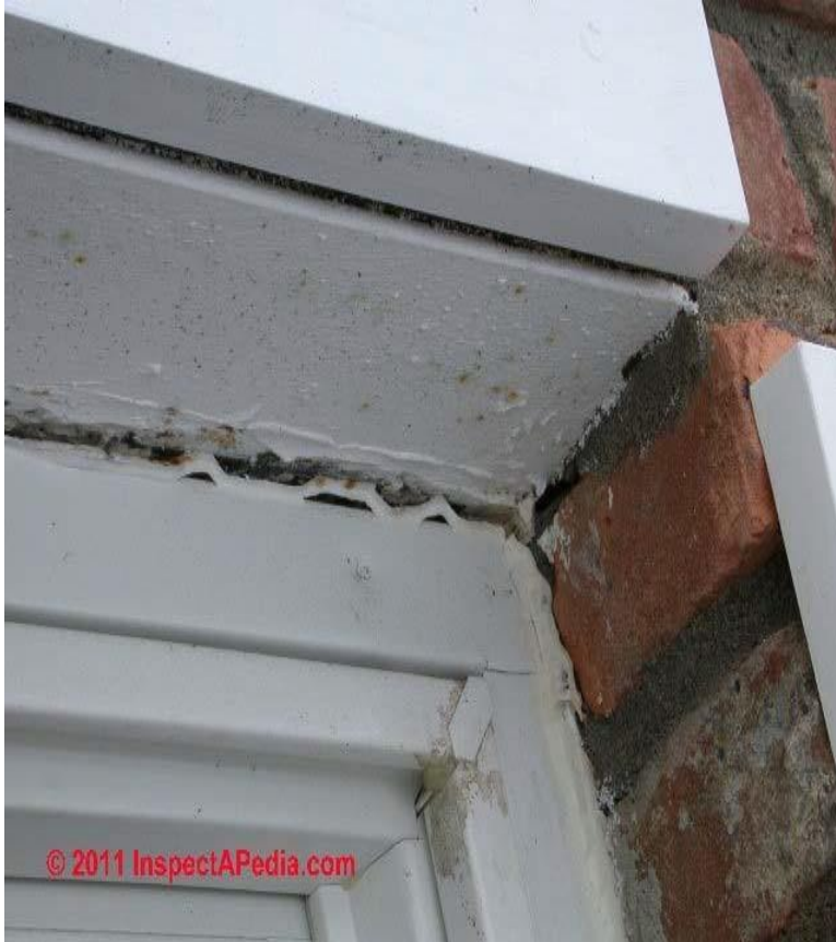
Shrinkage on drying
