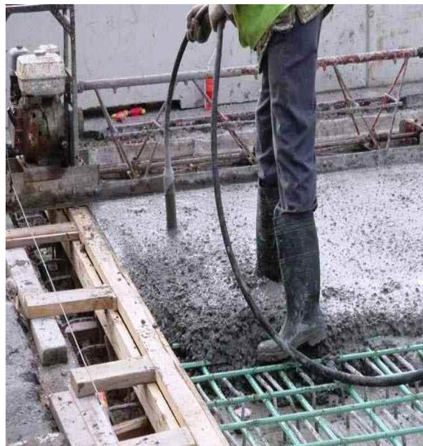
Figure 28: Compaction using vibrator
