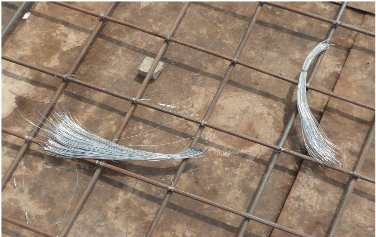
Figure 26: GI wire using in slab reinforcement binding
