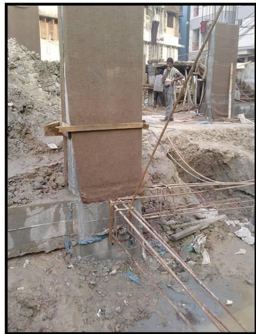
Figure 6: Curing of column
