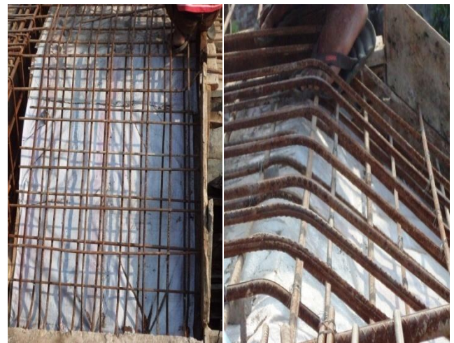
Figure 22: RCC of stair ( front & side view)
