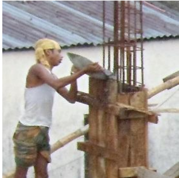
Figure 27: Concrete casting
