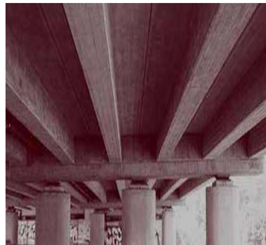
Figure 20: Joist/ ribbed slab
