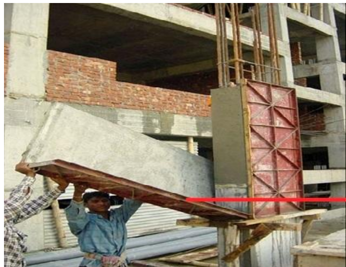
Figure 29: Removal of form work
