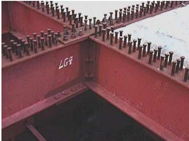
Figure 10: Steel Composite beam
