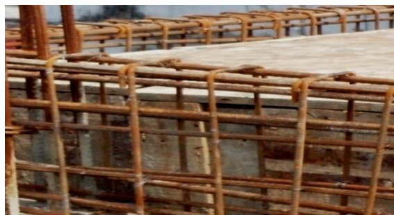
Figure 15: Hooking or bending of stirrups
