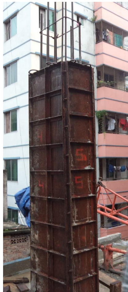
Figure 24: Shuttering
