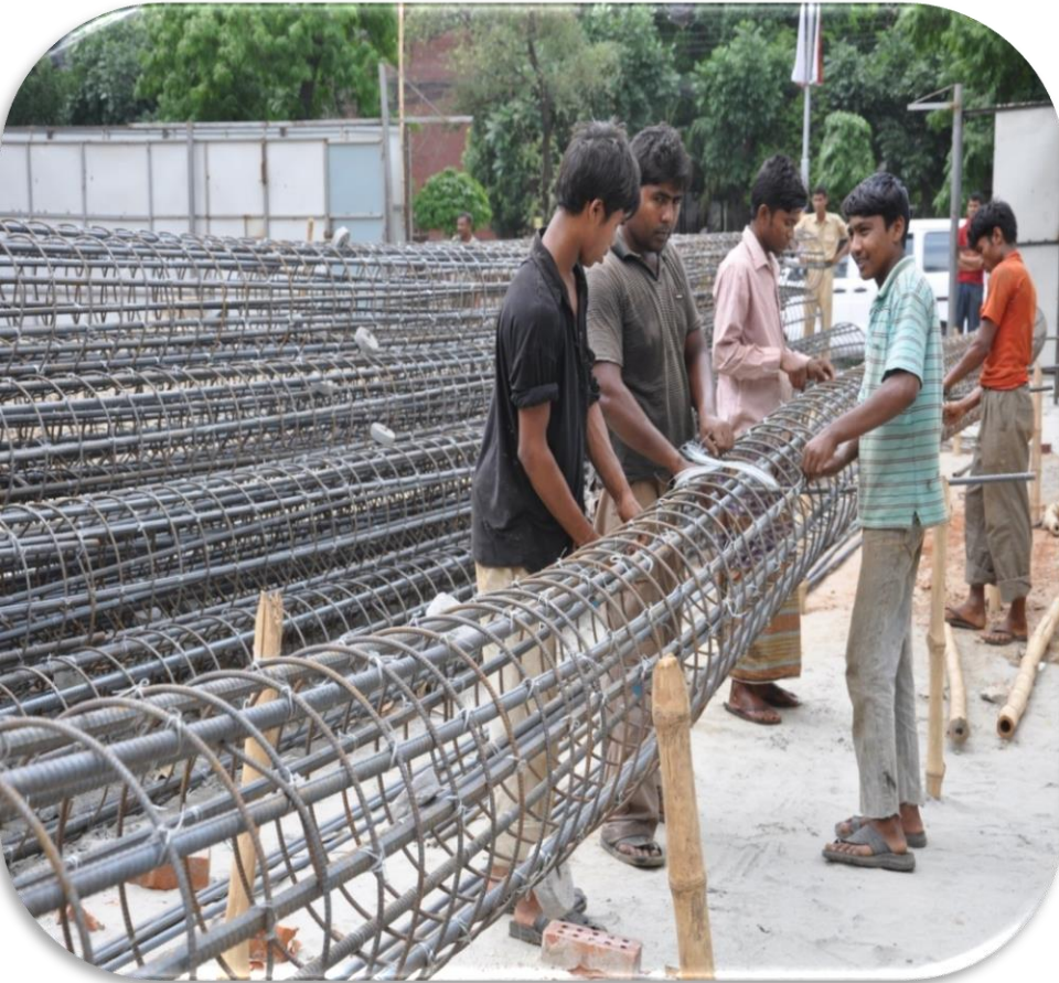
Circular shore piles' reinforcements are being constructed.
