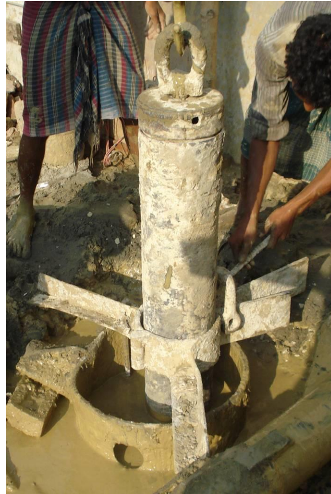
CLAMPING THE TREMIE PIPE
