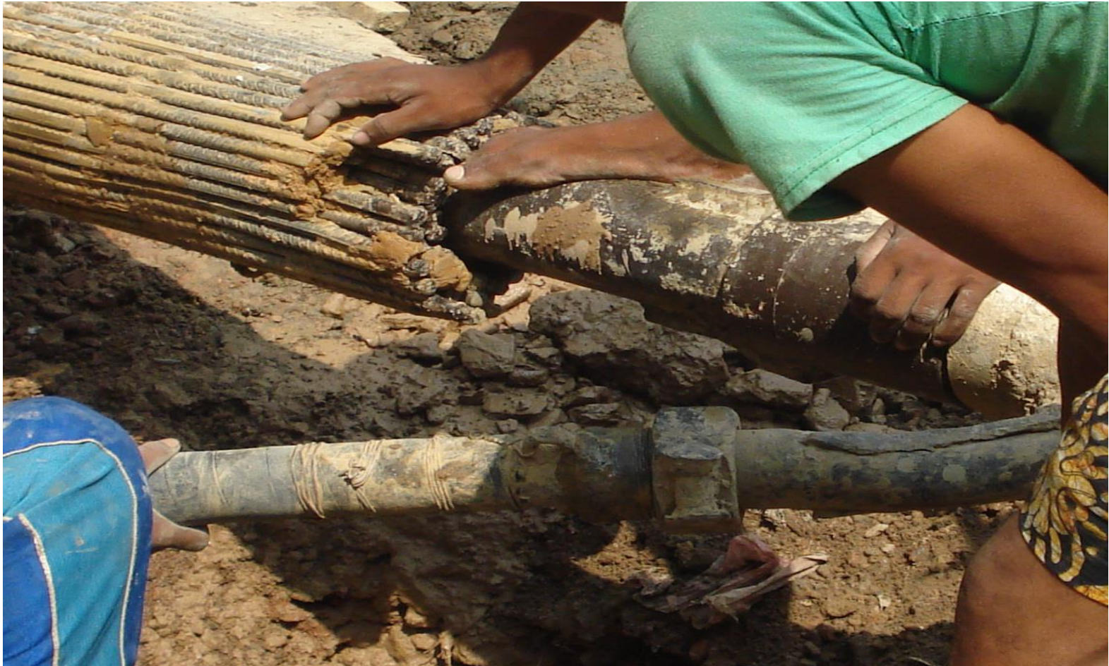
2. CONNECTING THE HOSE PIPE TO THE AUGER.
