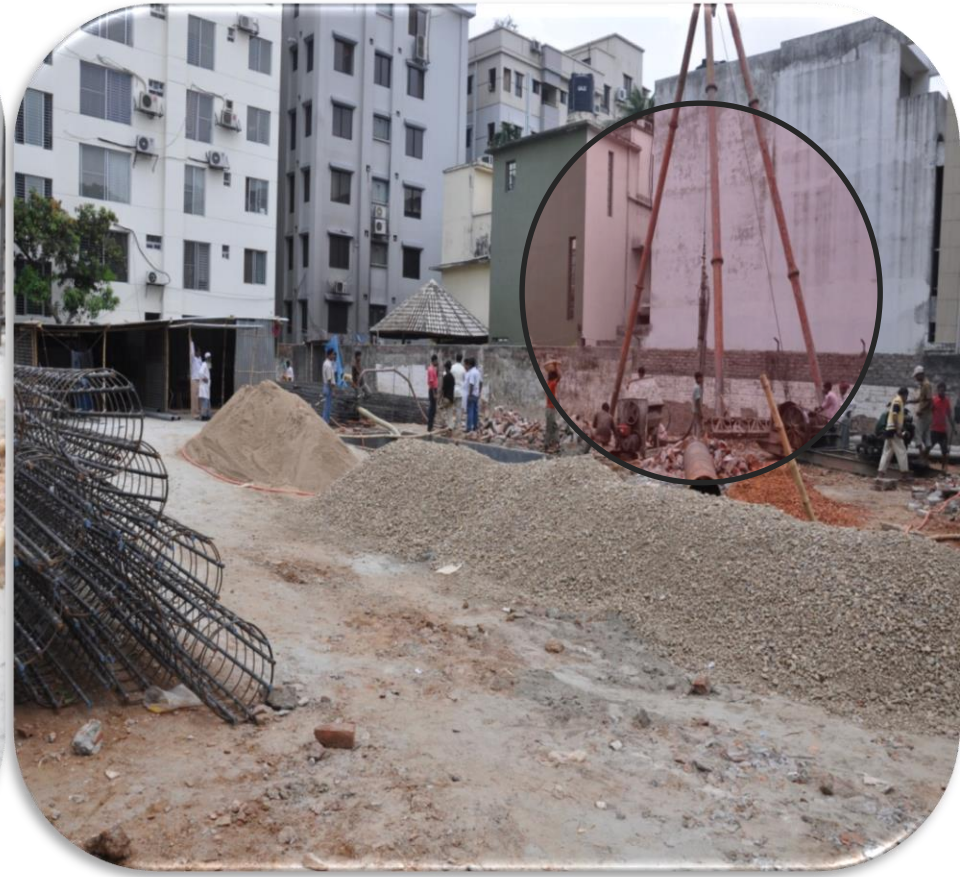
Boring work is going on.
