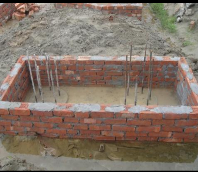
Pile cap for two piles
