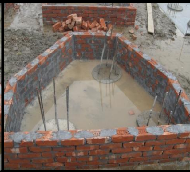
Pile cap for three piles
