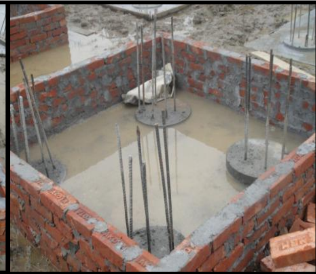
Pile cap for four piles
