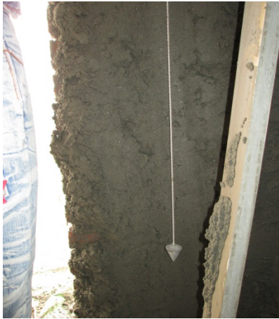
Fig: Leveling With Plumb Bob
