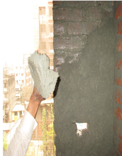
Fig: Covering with Cement Plaster
