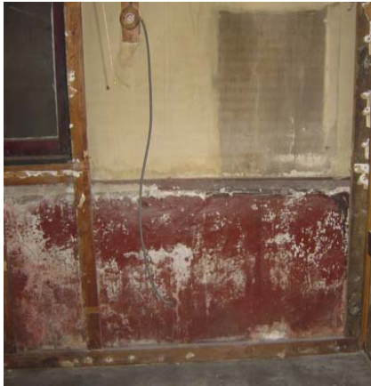
Fig: Efflorescence
