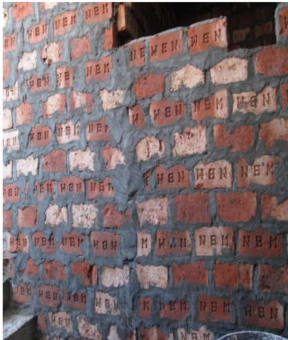
Fig: Preparing Surface
