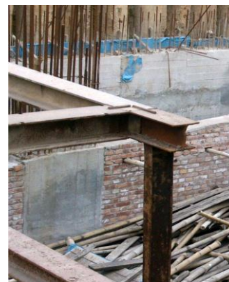
Figure 9: Vertical joist to support horizontal joists
