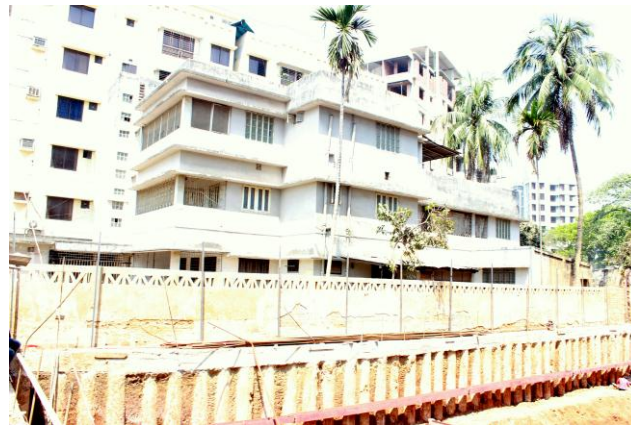
Figure 1: Shore Piling
