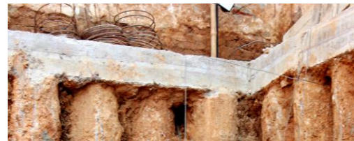
Figure 6: Tie Beam above the pile
