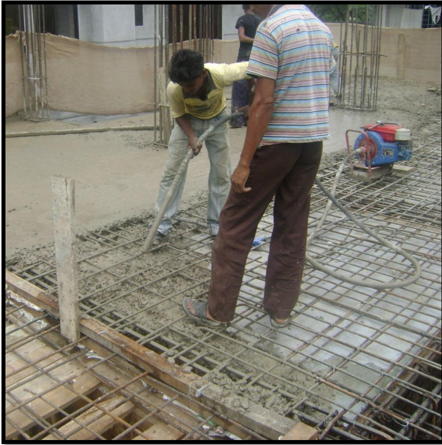
Use Of Vibrator
