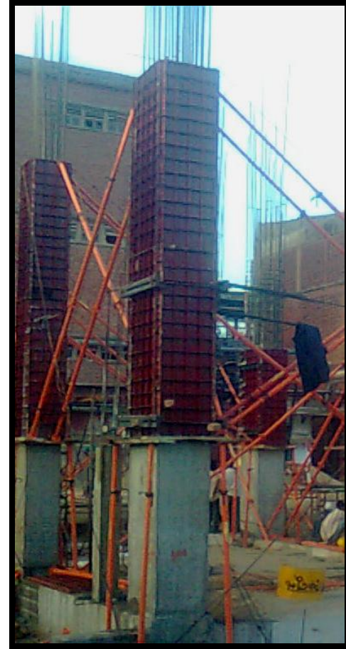
Steel Shuttering
