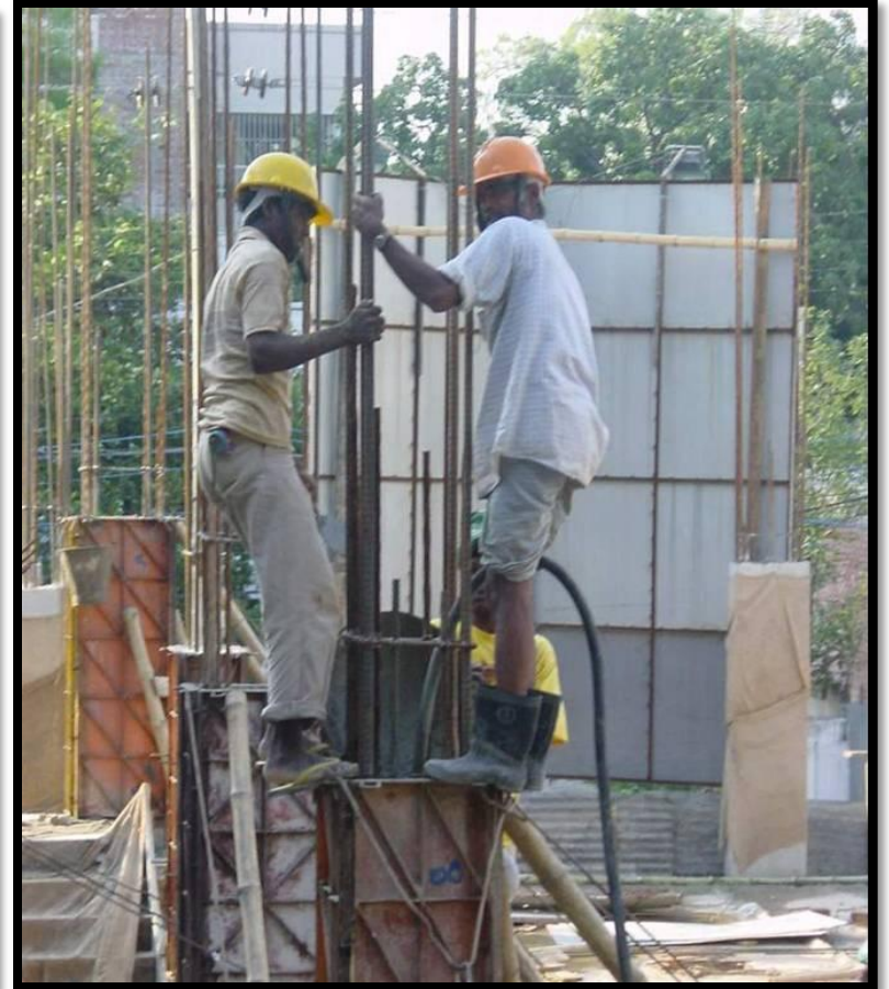
Use Of Vibrator
