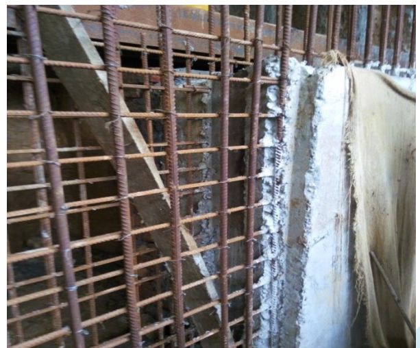
Fig 9: Position of Brick Wall, Felt Paper & Sand Fill
