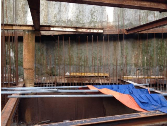
Fig 6: Ferrocement Layer on Shore Piles
