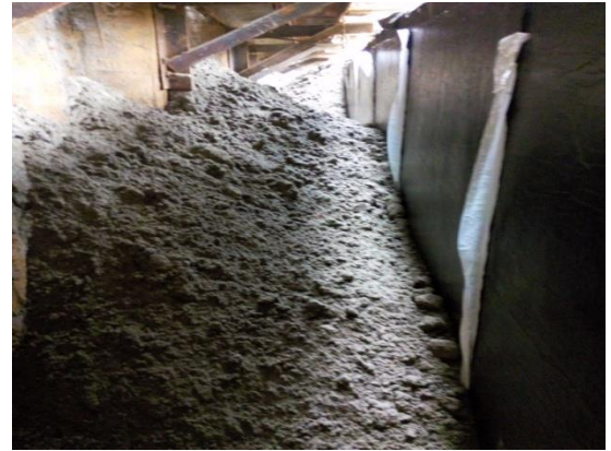
Fig 7: Bitumen Felt Layer on Exterior Brick wall
