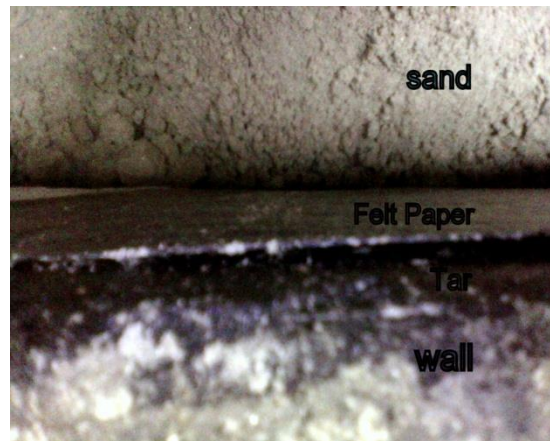
Fig 9: Position of Brick Wall, Felt Paper & Sand Fill
