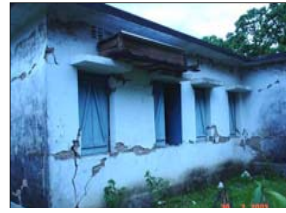
2003: Brick Masonry Building, Kolabunia
