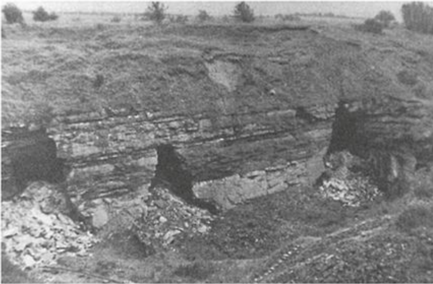
Figure 6.4 A quarry face showing abandoned room and pillar workings which are partially collapsed. The voids (rooms) have migrated upwards as the roofs have collapsed, and in one case (extreme left of photograph) only a thin layer of rock separates the void from the overlying soil. (Reproduced by kind permission of Messrs J.W.H. Ross & Co., Mining Engineers, Glasgow.)
