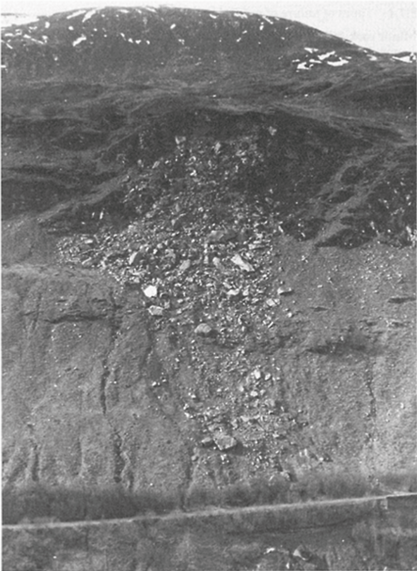
Figure 8.3 A major rock fall in the Scottish Highlands menacing the West Highland Railway. (British Geological Survey photograph, MNS1733(8), published by permission of the Director; NERC copyright.)
