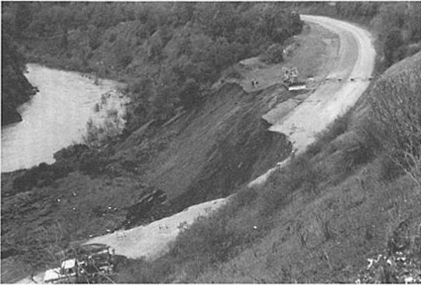
Figure 8.2 Slope failure at Sonoma County, California. (Reproduced by kind permission of California Division of Highways.)
