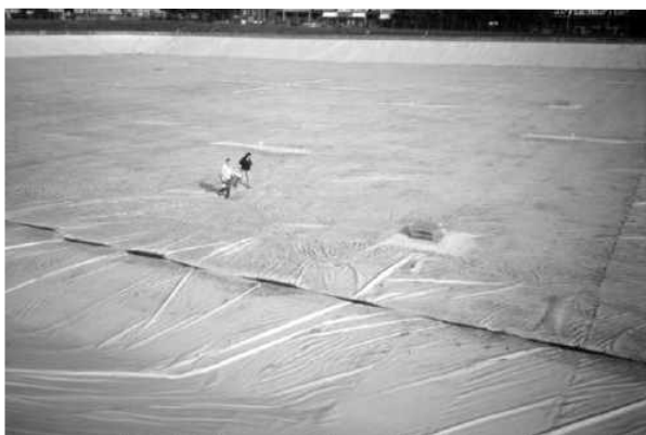
Figure 12.2: Preparing to sample stored drinking water from the access hatch of a floating cover on a distribution system reservoir
