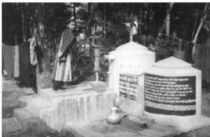
Figure 7.2: Typical Community Arsenic and Iron Removal Plant
