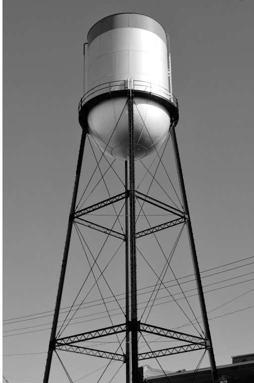
Figure 9.8: Elevated steel tank
