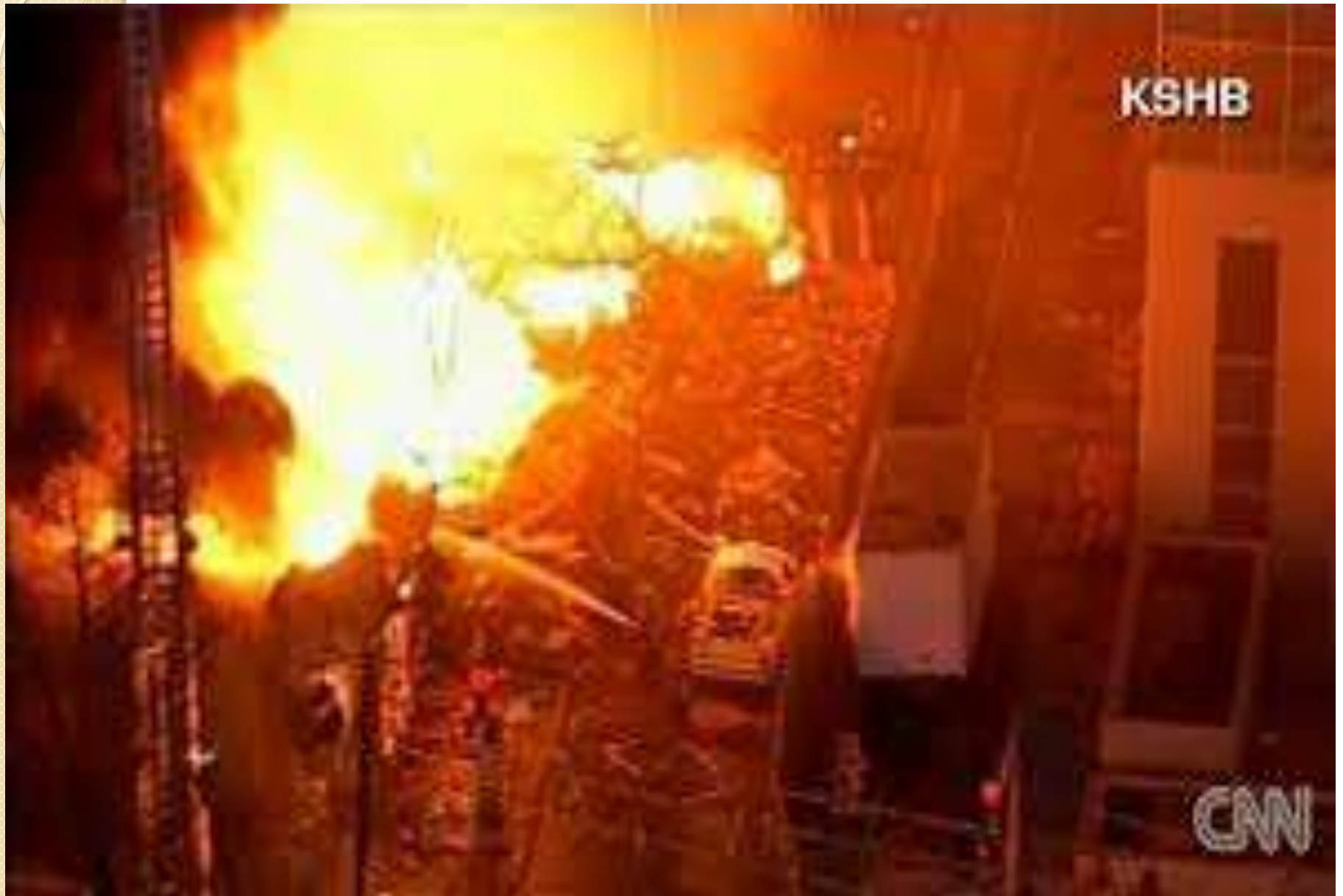
Fire during Construction Works
