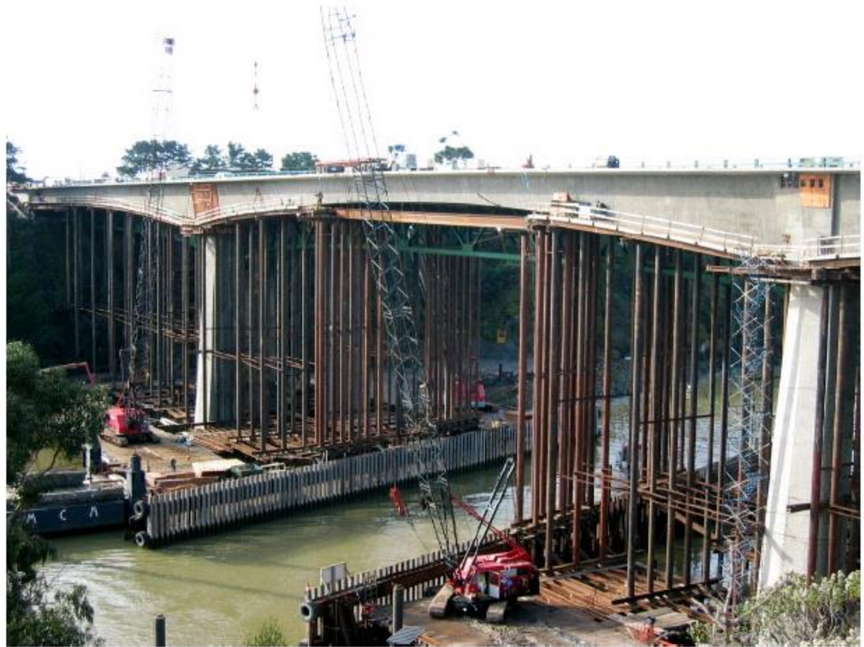
Figure 1.6 - Cast-In-Place Post-Tensioned Construction in California
