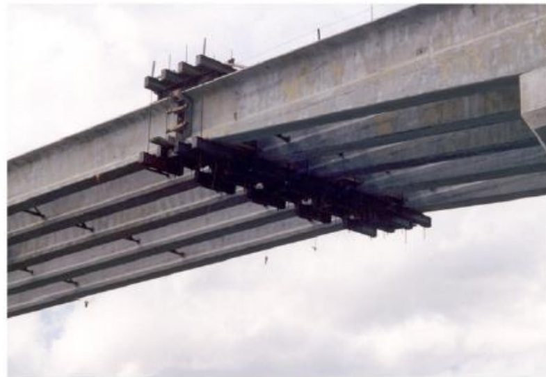
Figure 1.7 - Spliced Haunched I-Girder of Main Span Unit
