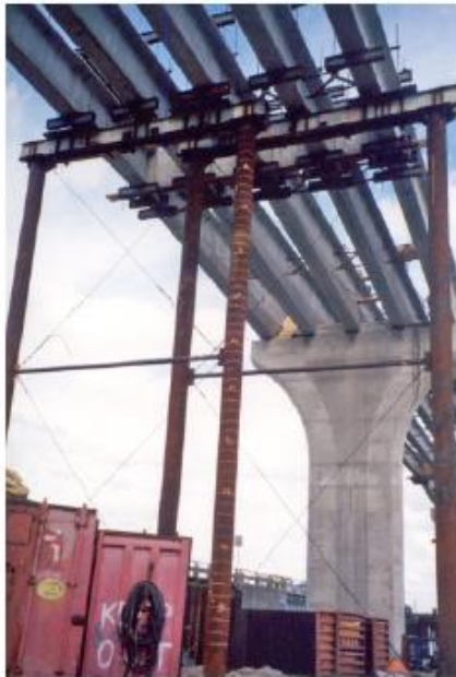
Figure 1.7 - Spliced Haunched I-Girder of Main Span Unit
