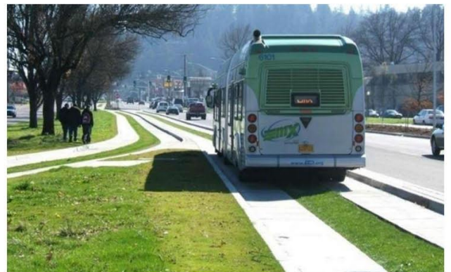
Use of Twin-Track system for Busway
