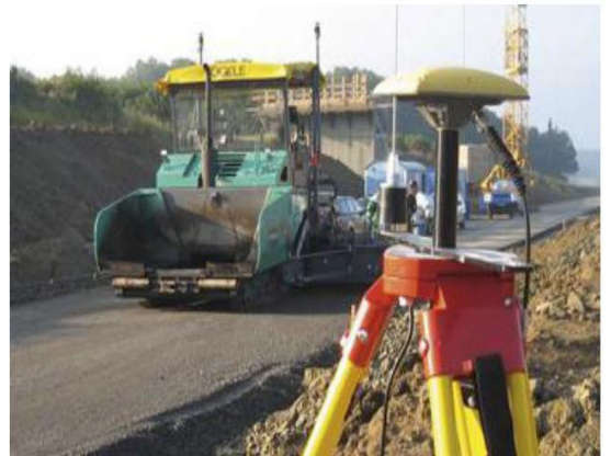
Paver with GPS (3D Positioning) System
