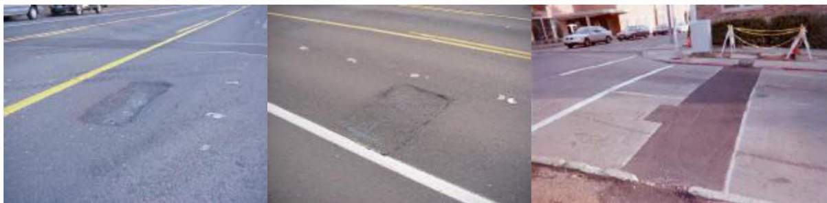
Failing patch
