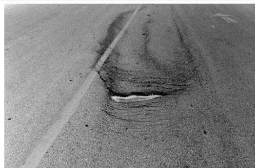
Slippage cracking
