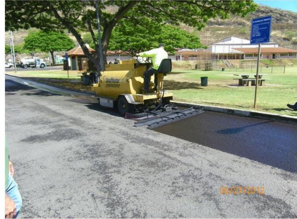
Slurry seal placement
