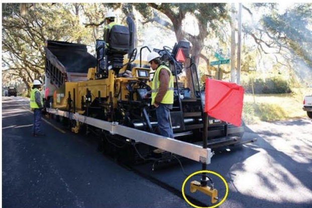
Paver with Sonic Levelling Device
