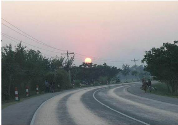
Channelized Traffic Causes Rutting Problems
