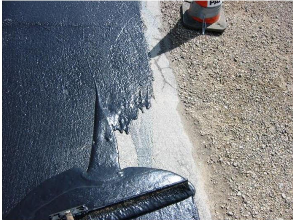
Slurry seal close-up.
