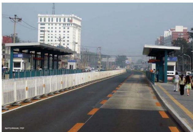
Use of Rigid Pavement at Bus Stoppage
