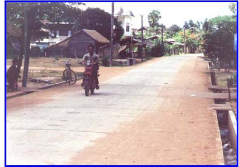
Image 3 – Bamboo Reinforced Concrete Paving
