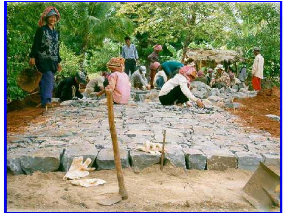
Image 2 – Dressed Stone Paving under Construction
