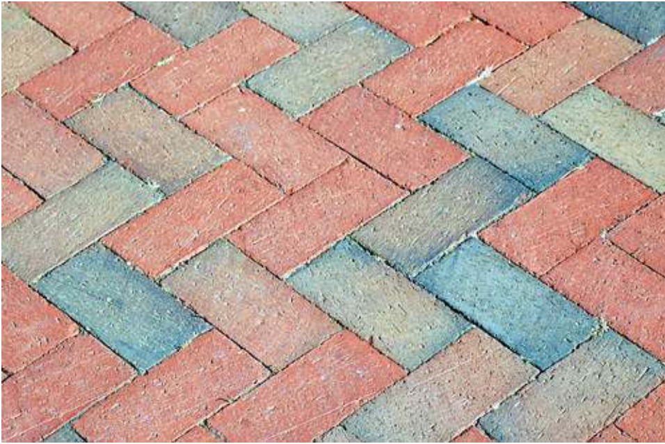
❖ Herringbone Bond Brick (HBB) on flat soling
