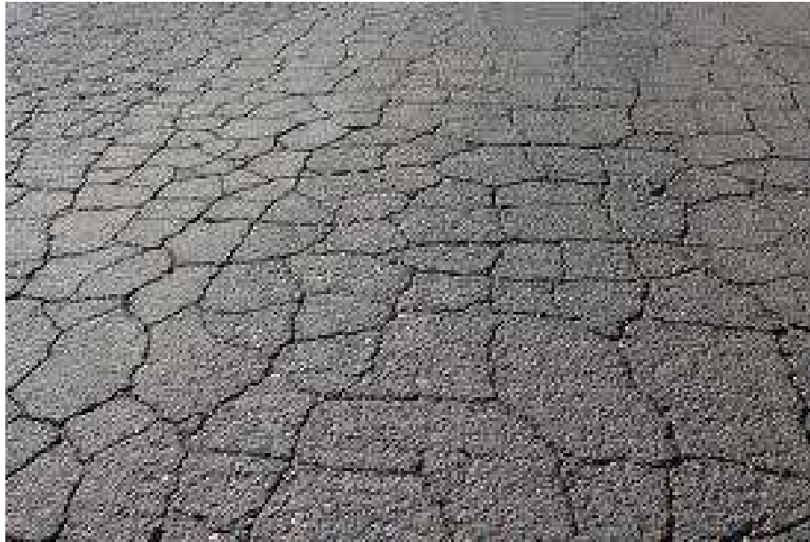
ALLIGATOR CRACK
