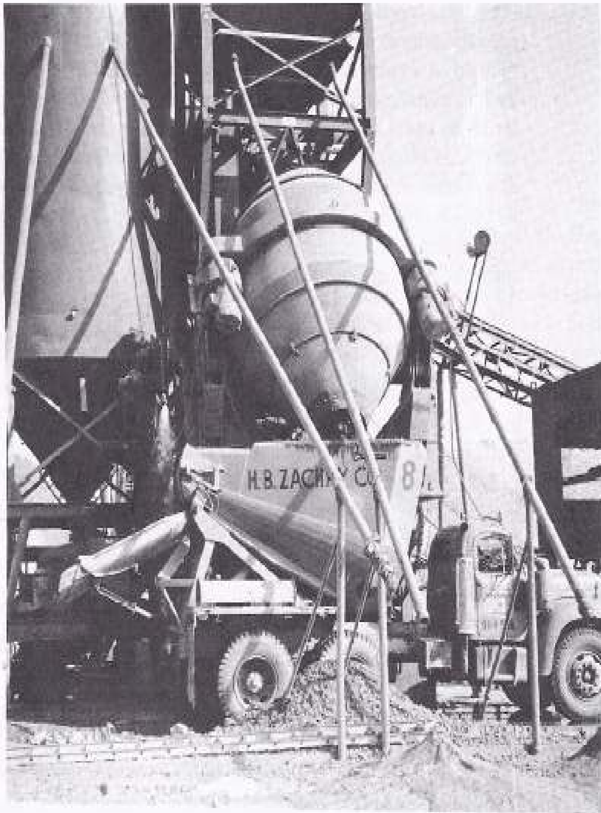
FIGURE 20-14 Tilting drum mixer discharging concrete into agitating body truck. (Courtesy Wire Reinforcement Institute.)
