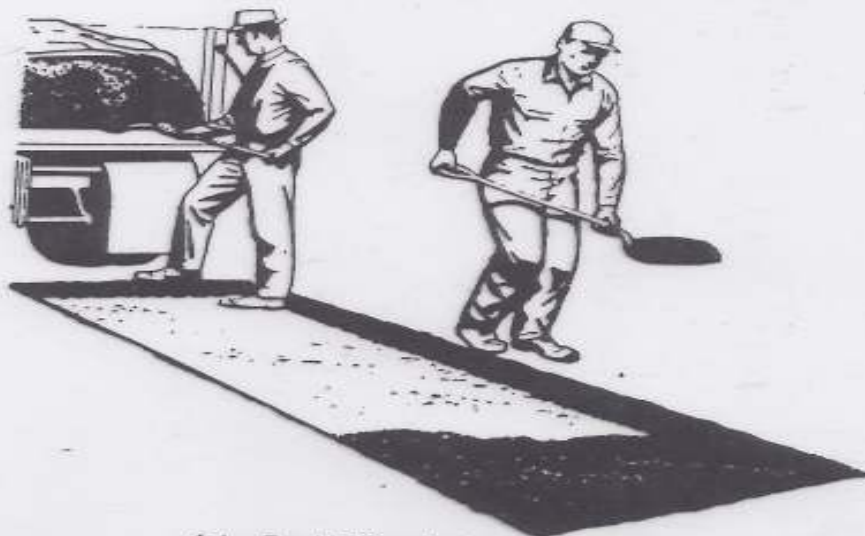
(c) Backfilling hole with plant-mix
