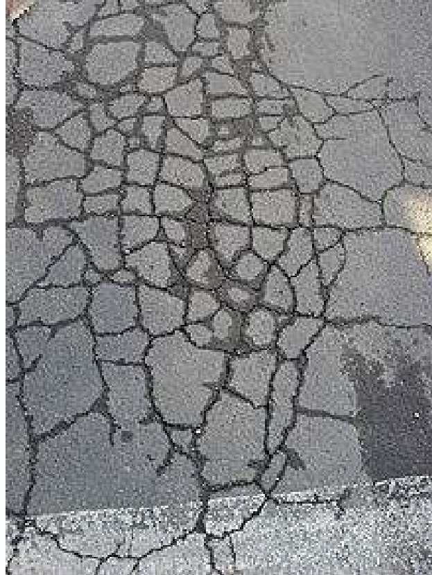
ALLIGATOR CRACK
