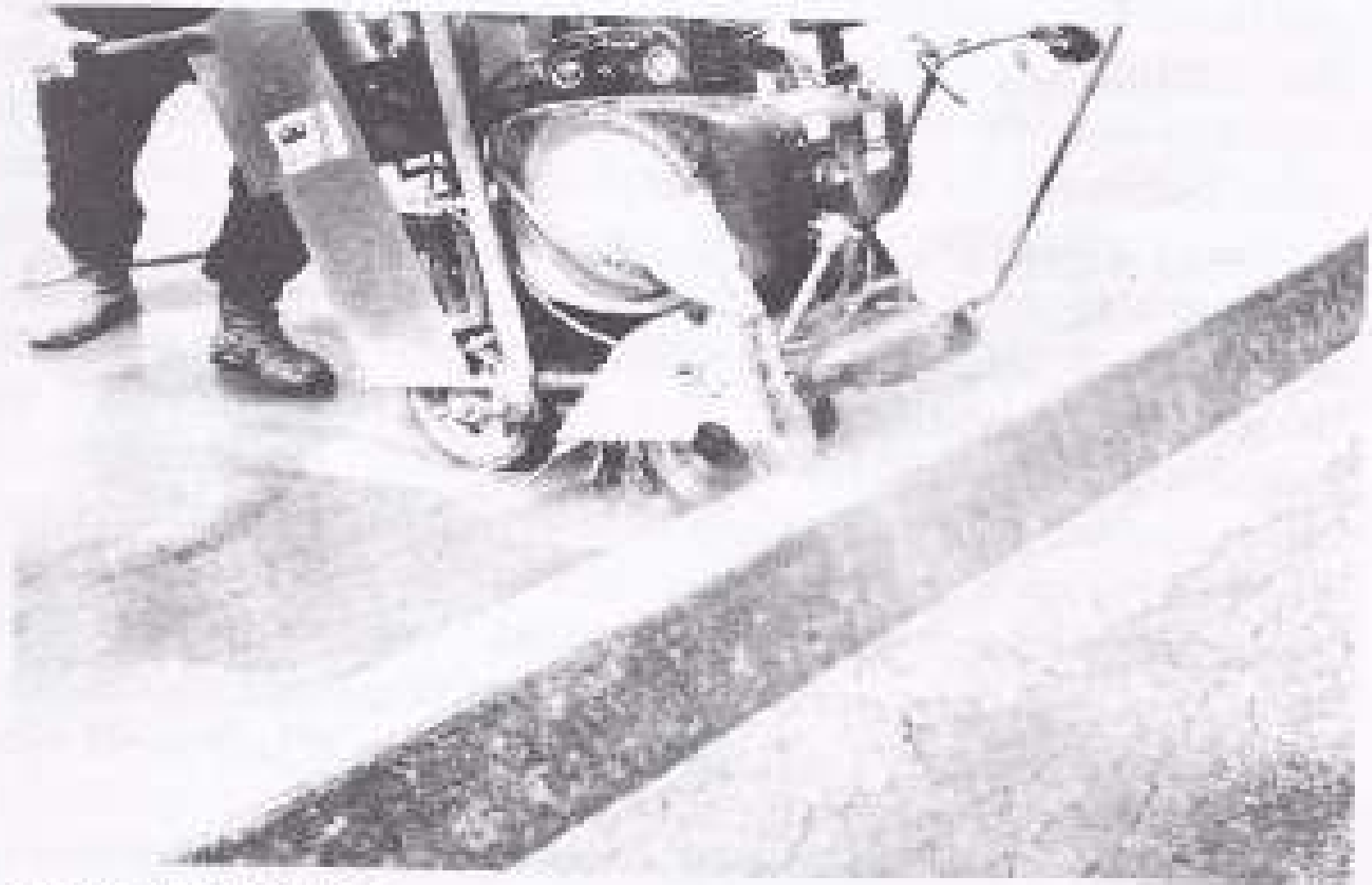
FIGURE 20-20 Concrete saw with a diamond blade cutting a pavement joint. (Courtesy Portland Cement Association.)
