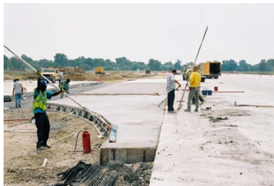
Figure 8.2 – A typical fillet construction operation
