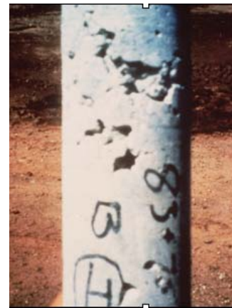
Figure 8.6 – Honeycombed concrete
