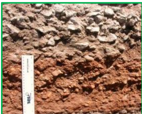
GCS base over natural gravel sub-base
