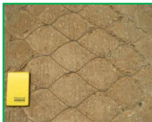
Geocell pavement 2 years after construction
