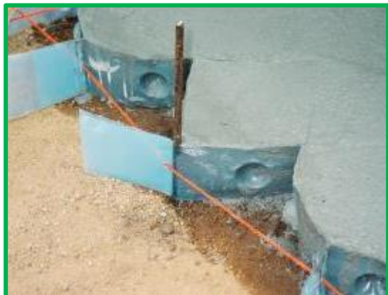
Geocells during construction
