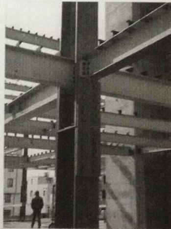
Column splice, Simple framing
