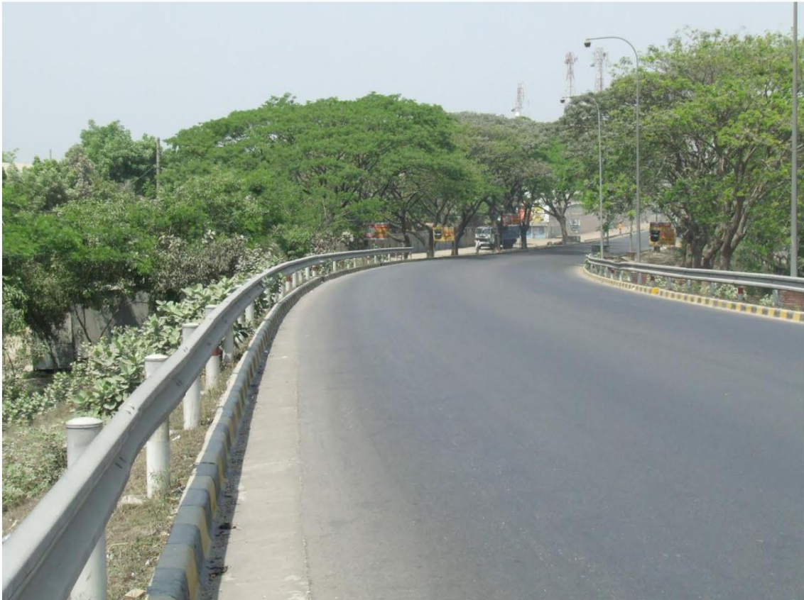
Road Side Continuous W-Beam Safety Barrier
