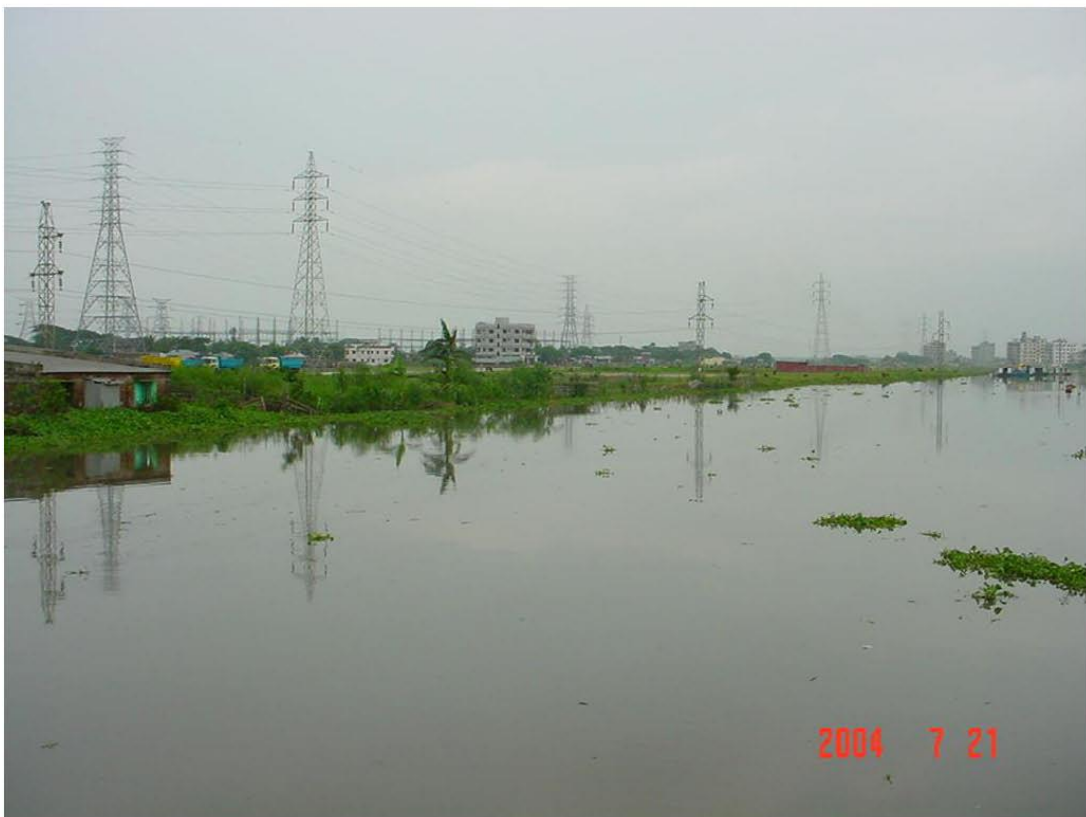
Electric Transmission Line
