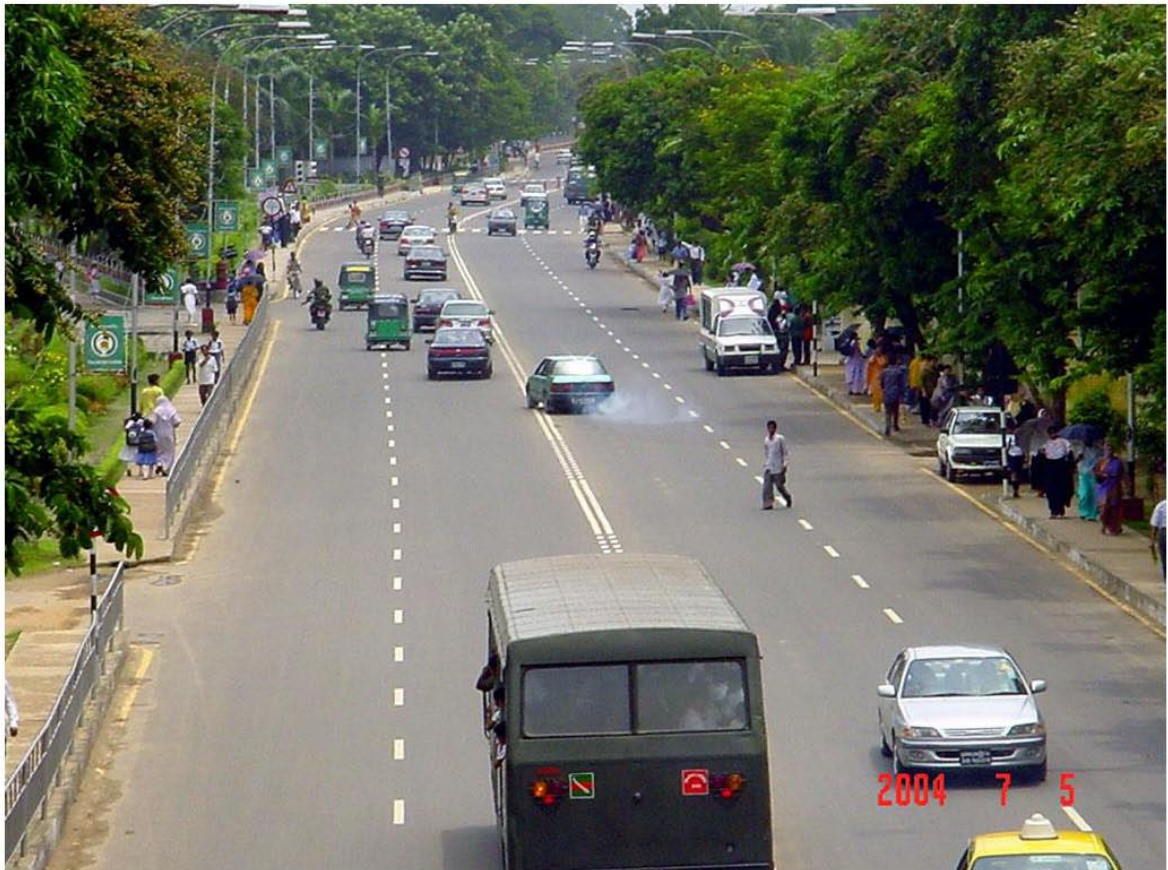
Road with Channelized Footpath and Appropriate Carriageway Signs and Markings
