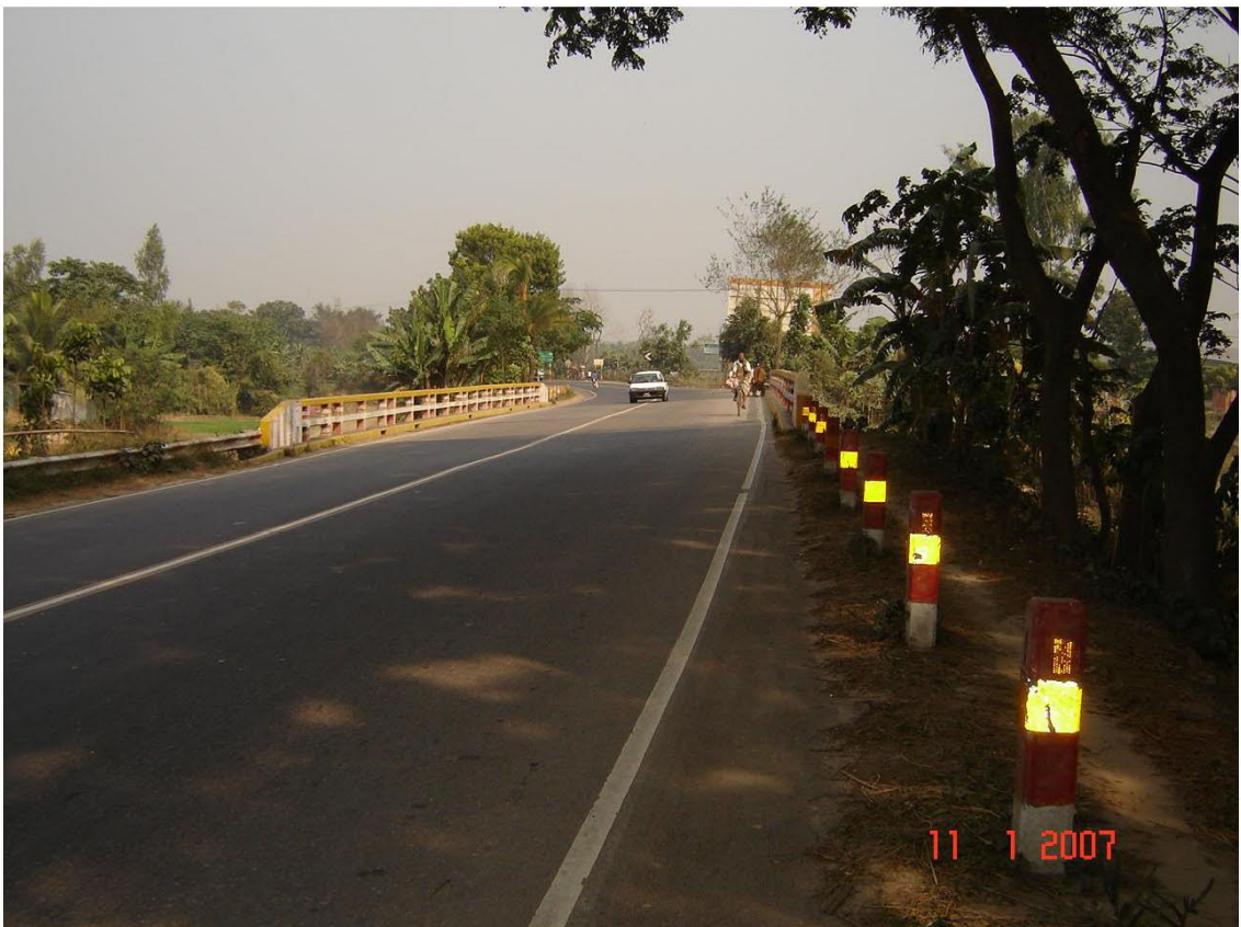
Guide Posts with Retro-Reflective Object Markings to Aid Nighttime Driving
