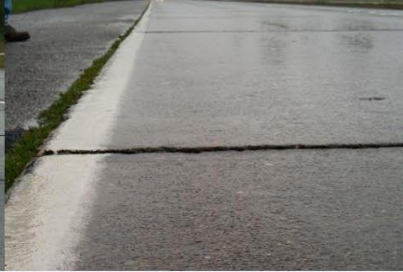
Figure 2: Faulting close-up.
