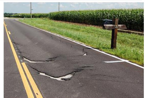
Slippage cracking
