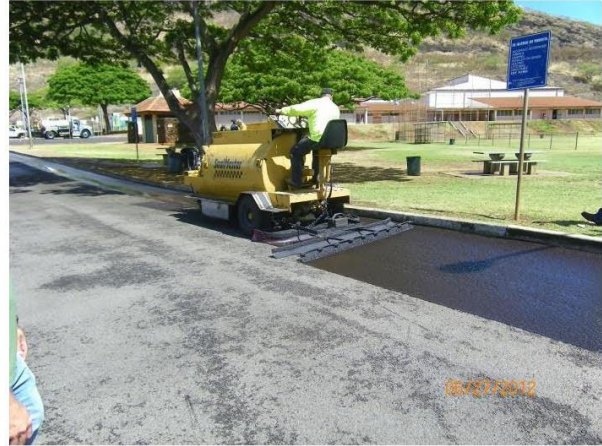
Slurry seal placement
