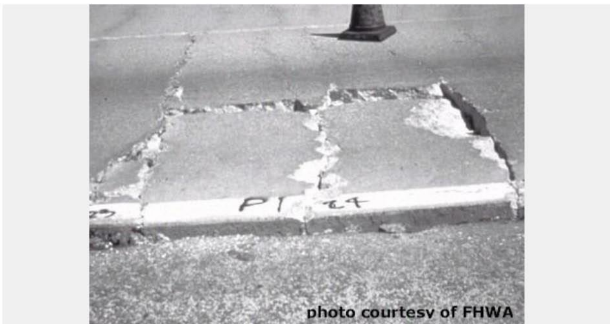
Figure 1: Severe punchout.
