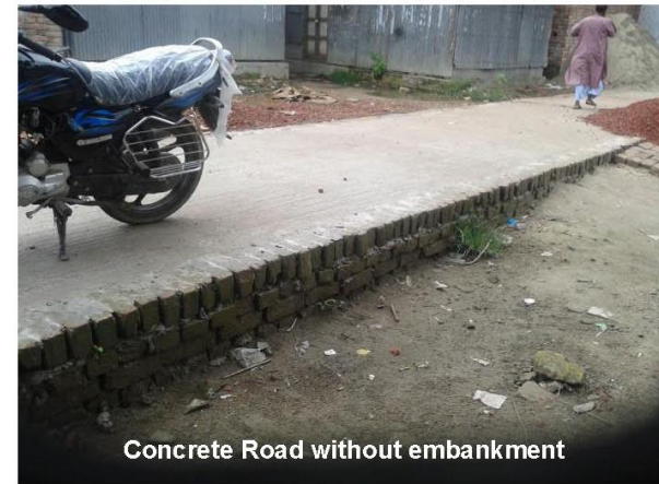
Concrete road at tight by-lane (Roller inaccessible)
