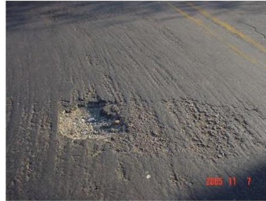
Developing pothole
