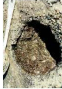
Stripping at bottom of hole
