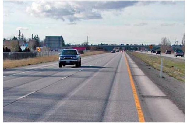
Channelized Traffic Causes Rutting Problems
