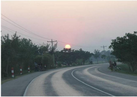
Channelized Traffic Causes Rutting Problems
