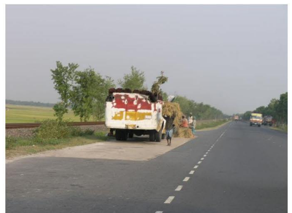
Use of Rigid Pavement at Waiting Area
