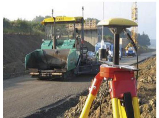
Paver with GPS (3D Positioning) System
