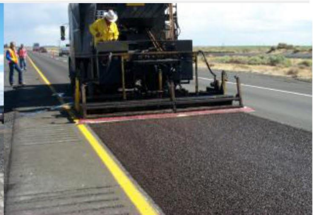
Figure 2: Micro-surfacing placement.
