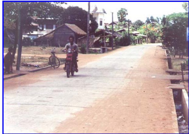
Image 3 – Bamboo Reinforced Concrete Paving
