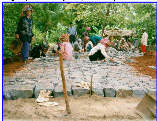
Image 2 – Dressed Stone Paving under Construction
