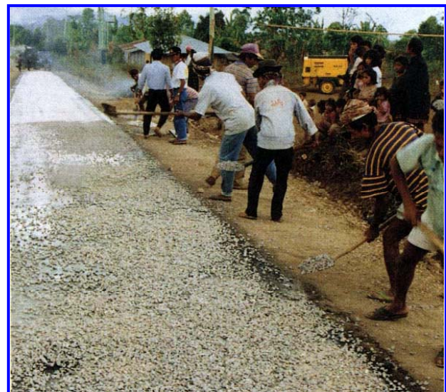
Image 4 – Hand Laid Bituminous Surface Dressing
