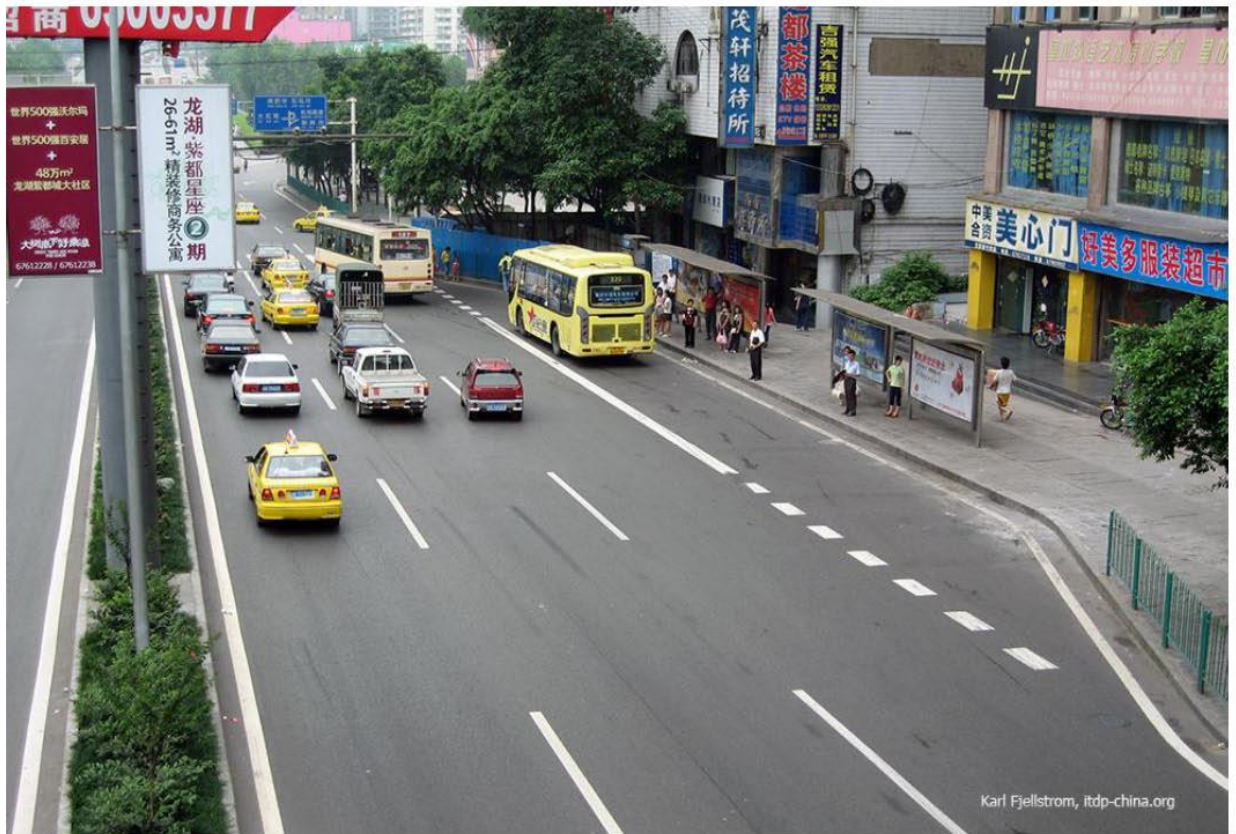
Road with Nice Bus Lay-by/Pullout
