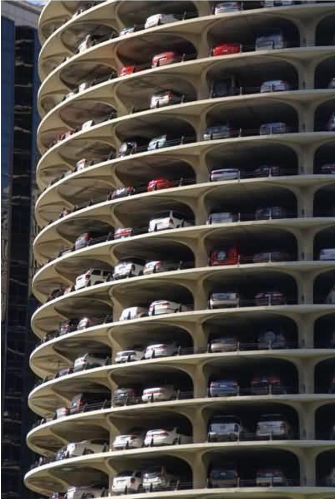
Multi-storied off street parkings
