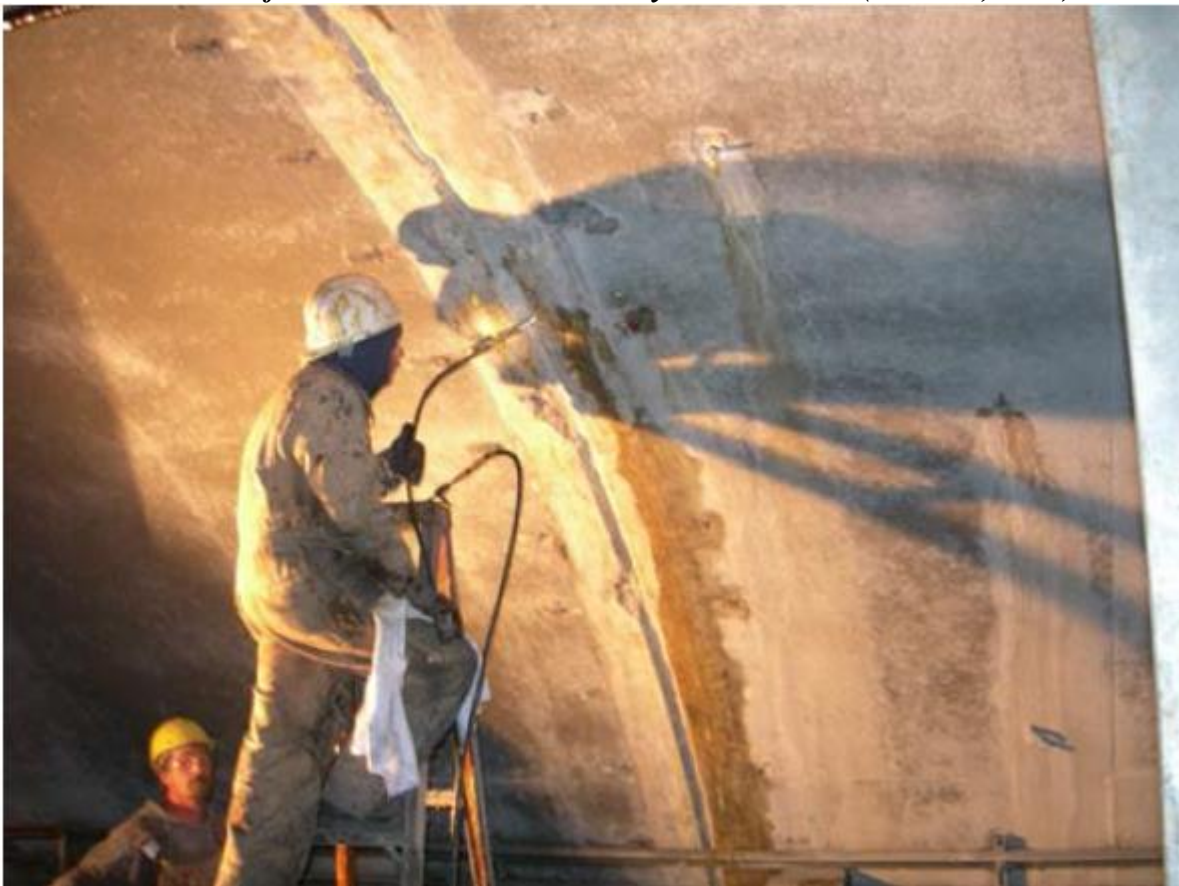
Leak Injection, Tuscarora Tunnel PA Turnpike
