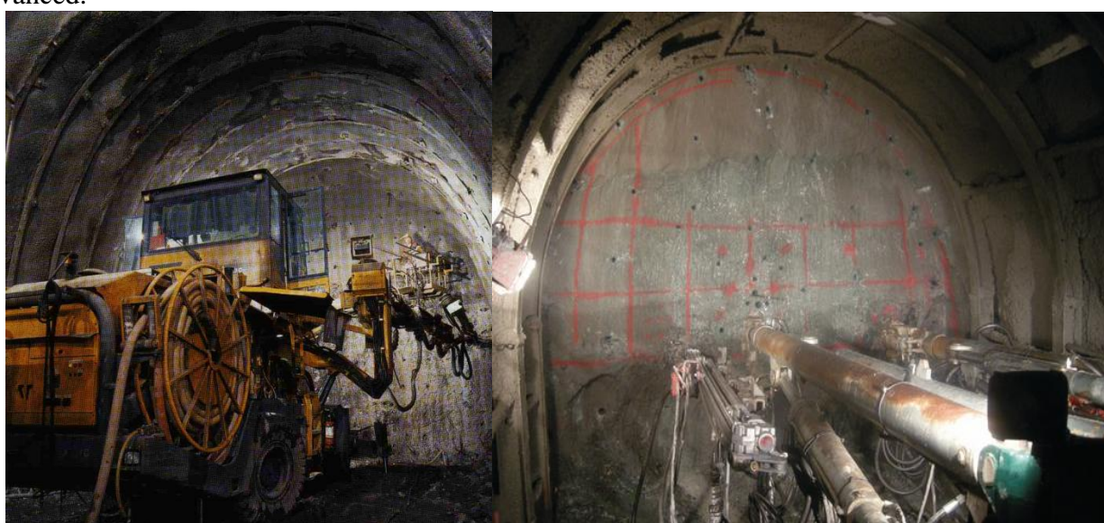
Figure.75 - Vehicle with bore jumbos to drill shotholes for a later blast
