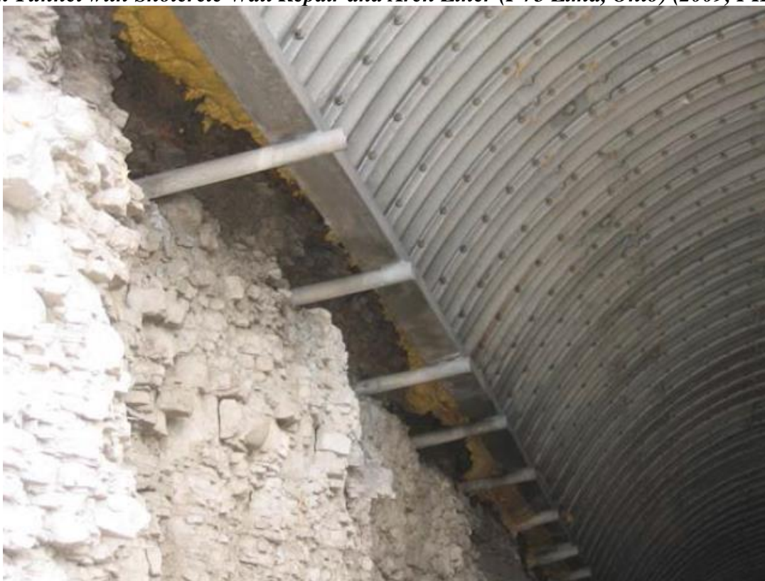
Rock Bolts (Dowels) Supporting Liner, I-75 Lima, Ohio Underpass (2009, FHWA)
