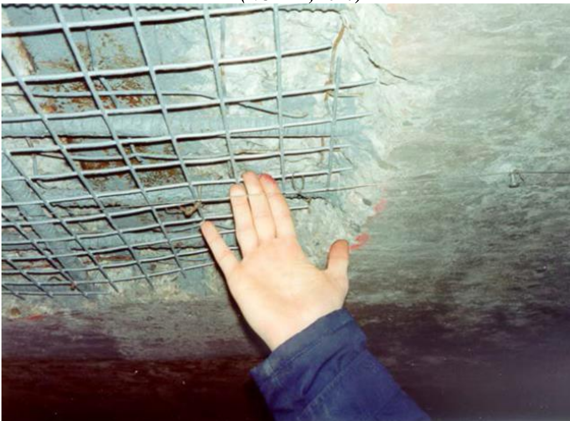
Reinforcing Steel for Repair, Sumner Tunnel- Boston, MA
