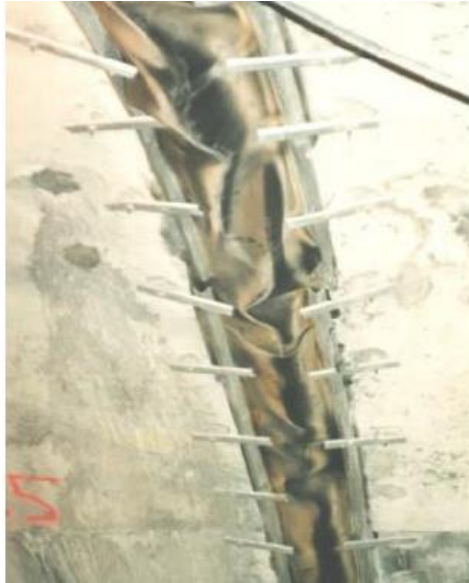
Temporary Drainage Systems Comprised of Neoprene Rubber Troughs and 25 mm (1") Aluminum Channels (FHWA, 2005)
