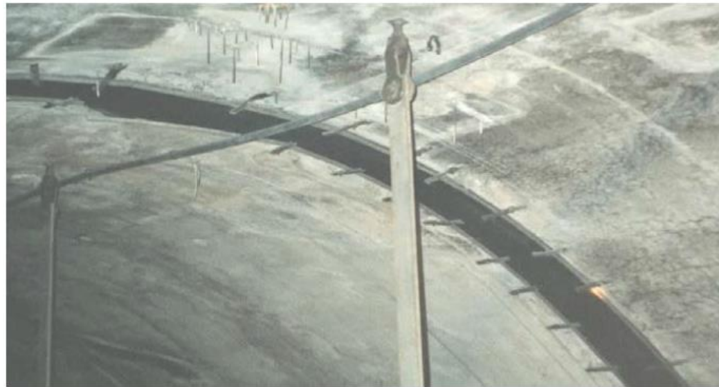
Temporary Drainage Systems Comprised of Neoprene Rubber Troughs and 25 mm (1") Aluminum Channels (FHWA, 2005)
