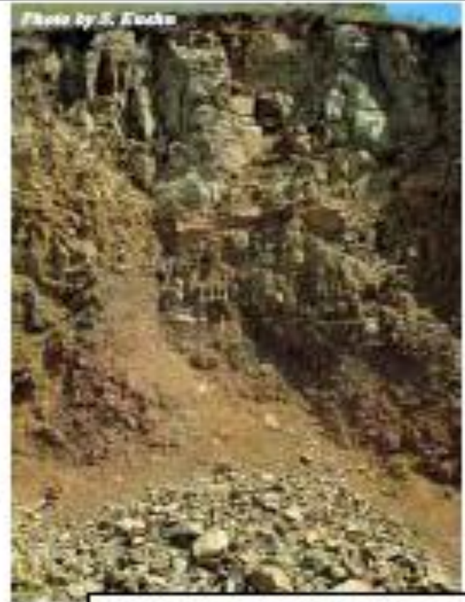
Small rockfall in a road cut in the Blue Mountains of Oregon
