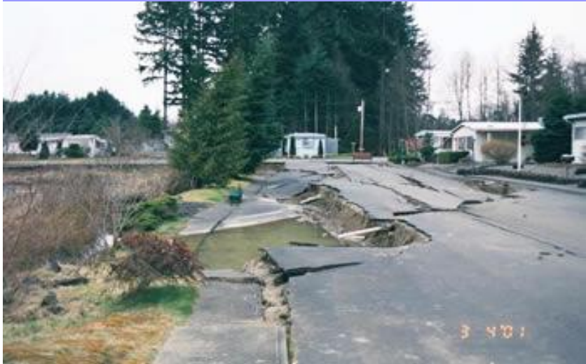
occurs when the soil mass spreads laterally and this spreading comes with tensional cracks in the soil mass.
