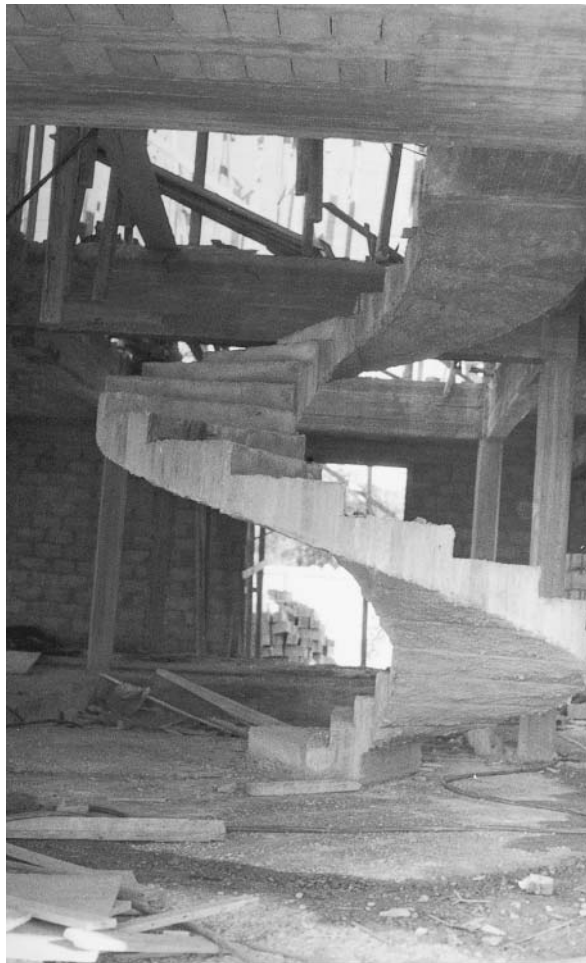
Reinforced concrete helical staircase.
