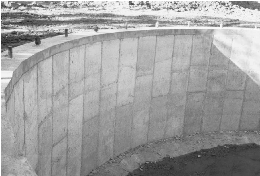
Reinforced concrete retaining wall.
