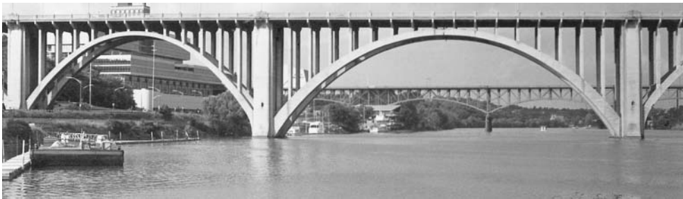
Concrete bridge, Knoxville, Tennessee.
