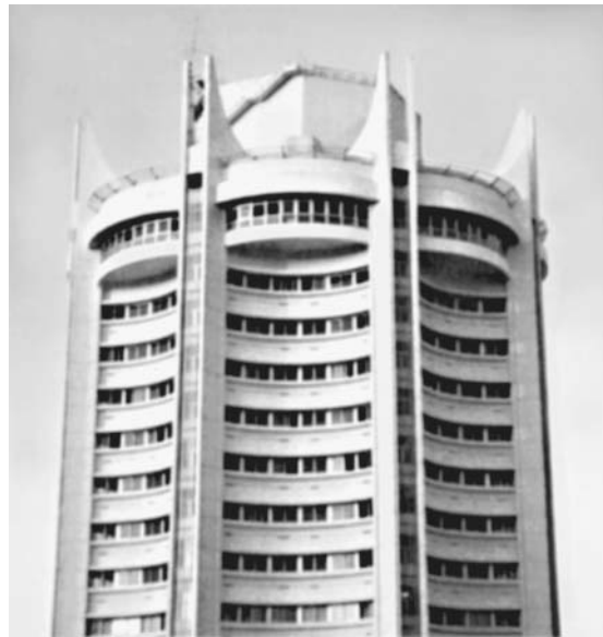
Circular beams in an office building.
