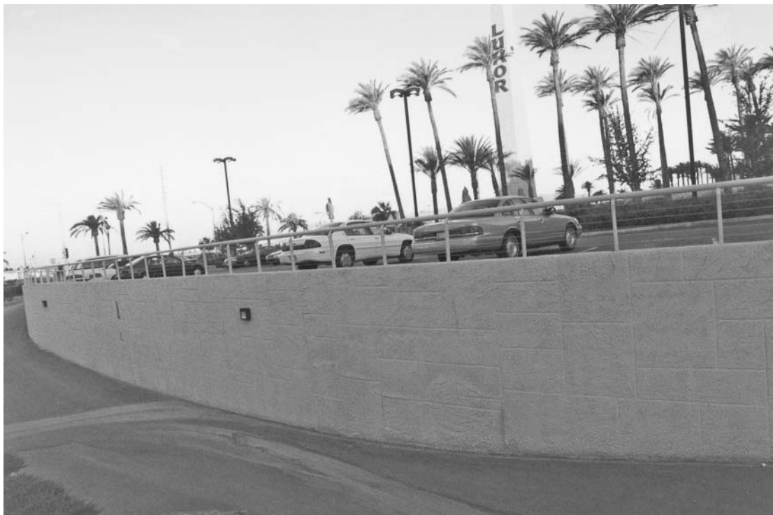
Retaining wall in a parking area.
