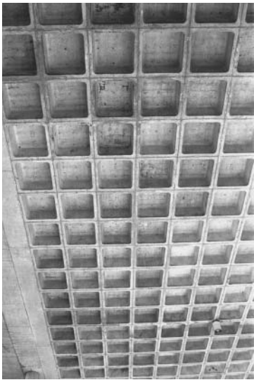
Waffle slab (looking upward).
