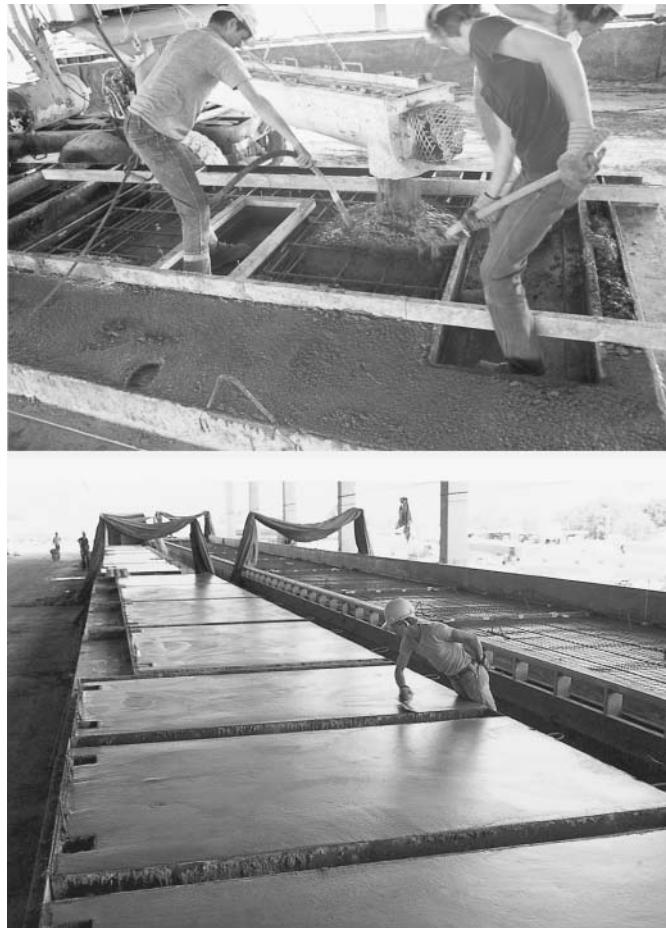
Casting and finishing precast concrete wall panels.
