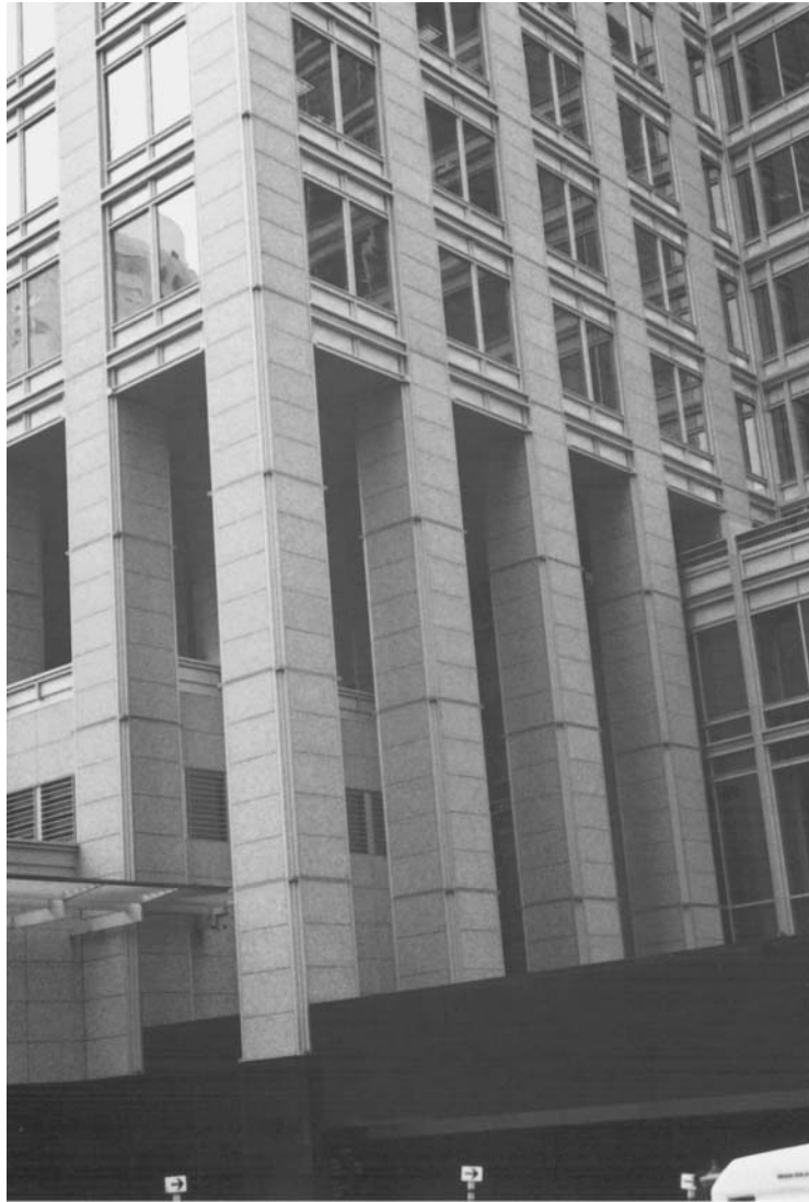
Long columns in an office building
