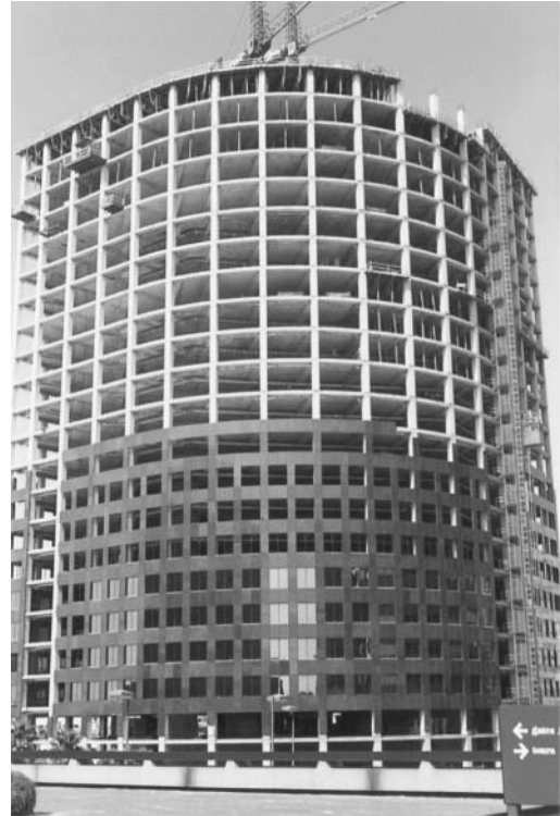
Office building under construction, New Orleans, Louisiana.
