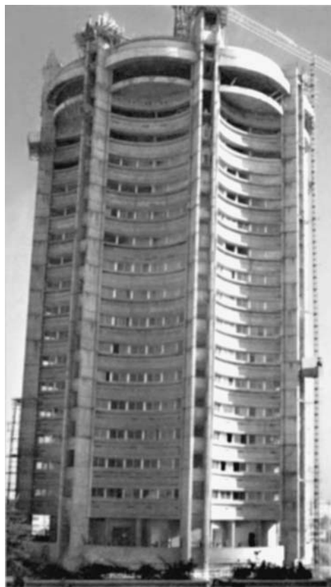
Curved beams in an office building.
