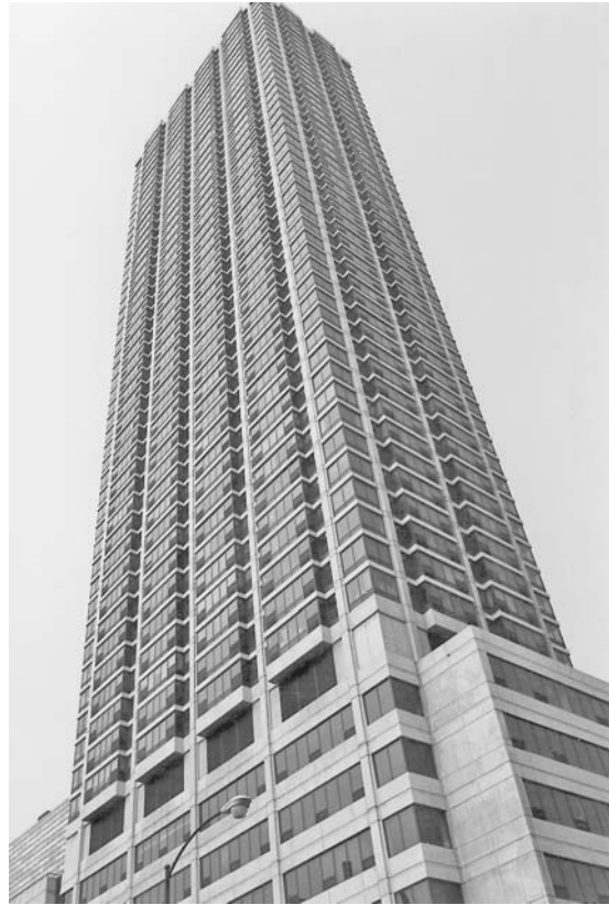
High-rise building, Chicago, Illinois.
