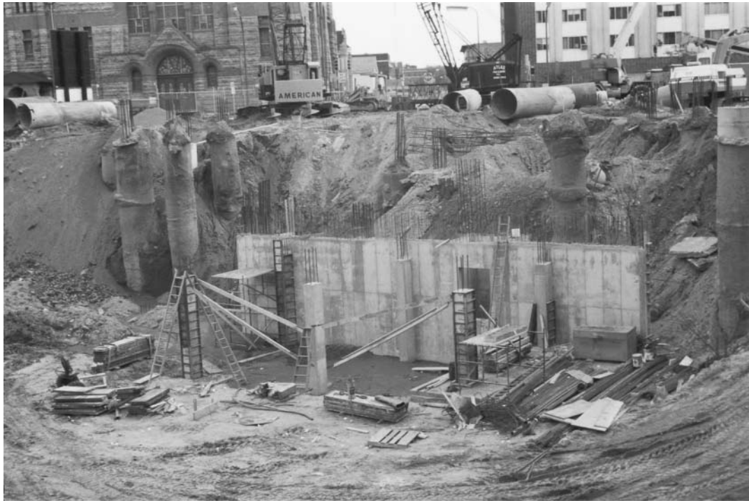
Wall and column footings, partly covered.
