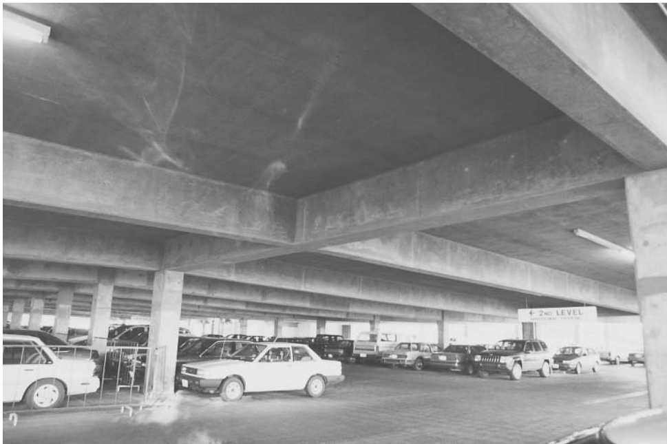
Slab on beams.
