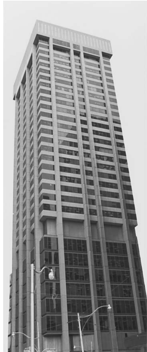
Columns in a high-rise building, Toronto, Canada.
