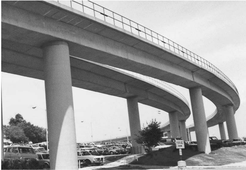
Curved-beam bridge, Washington, D.C.
