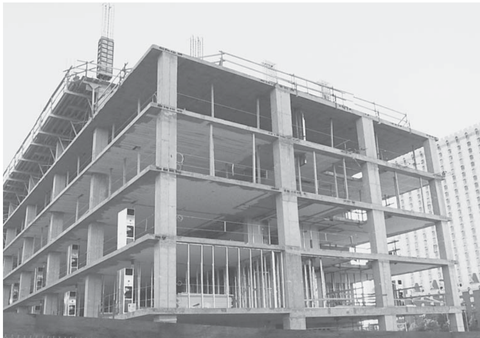
Flat-plate floor system.
