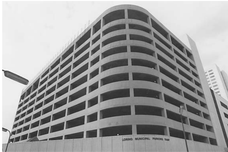
Reinforced concrete parking structure, Minneapolis, Minnesota.
