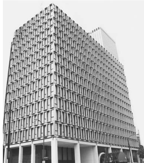
Office building, Chicago, Illinois.
