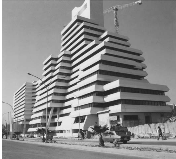
Reinforced concrete office building, Amman, Jordan.
