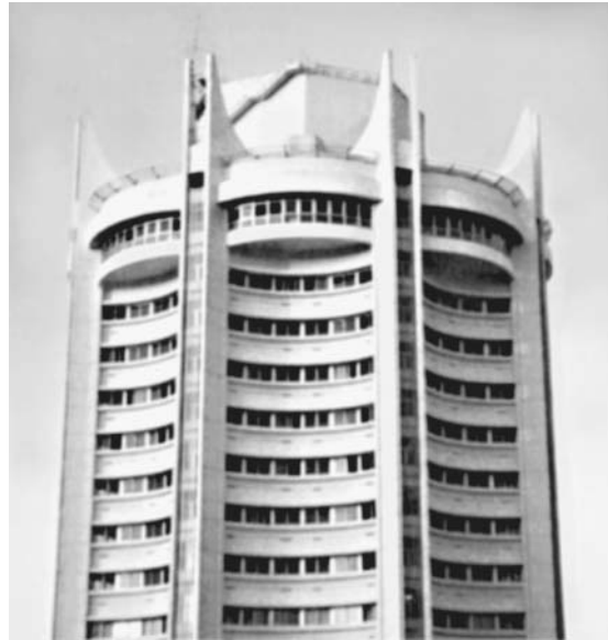
Circular beams in an office building.
