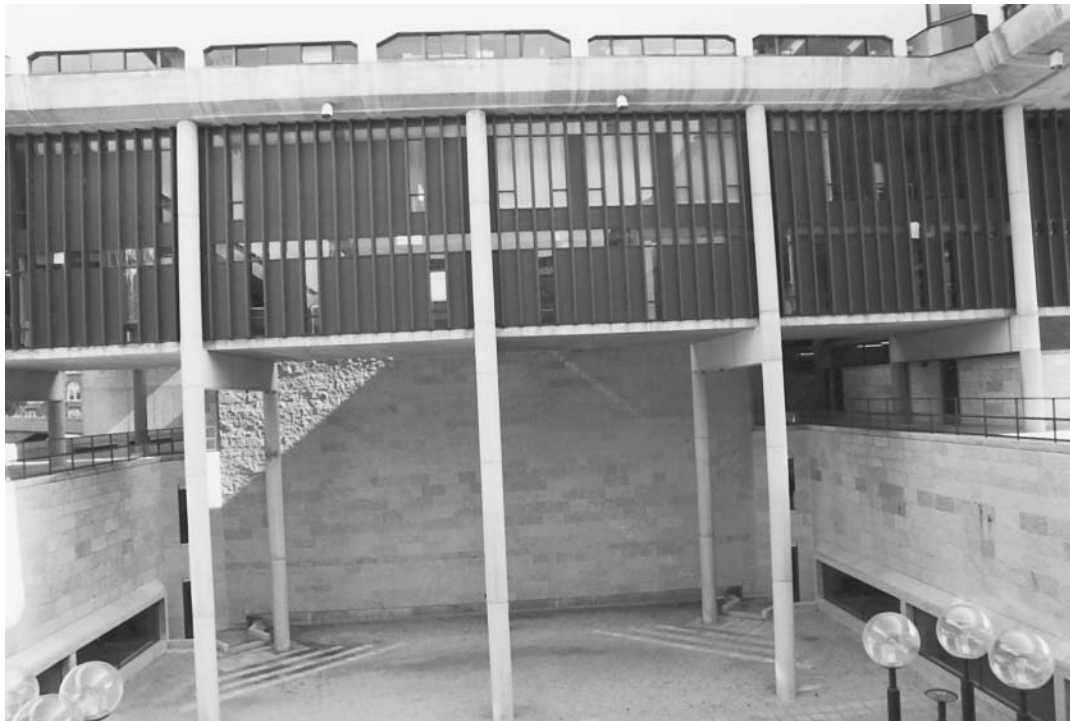
Columns, University of Wisconsin, Madison, Wisconsin.
