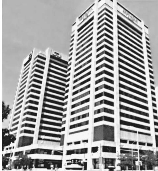
90° V-shape beams, London, Ontario, Canada.
