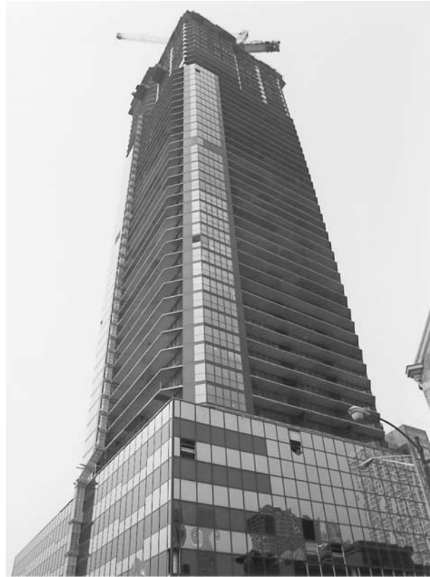
Office building under construction, Chicago, Illinois.
