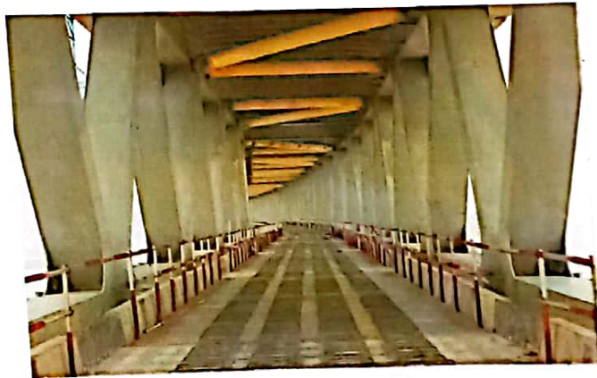
Fig : Rail track of Padma bridge
