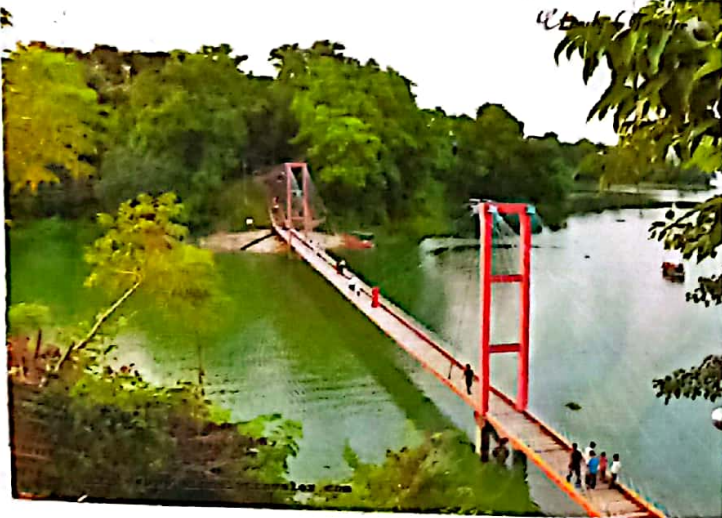
Figure: Hanging Bridge - Rangamati
