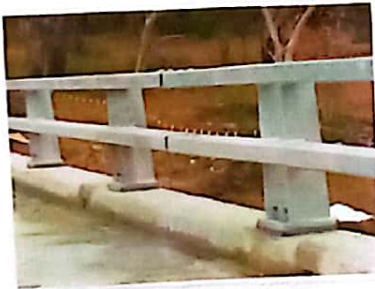
Fig : Curb of a bridge
