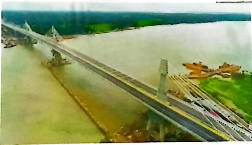
Figure: Shah Amanat Bridge - Chattogram.
