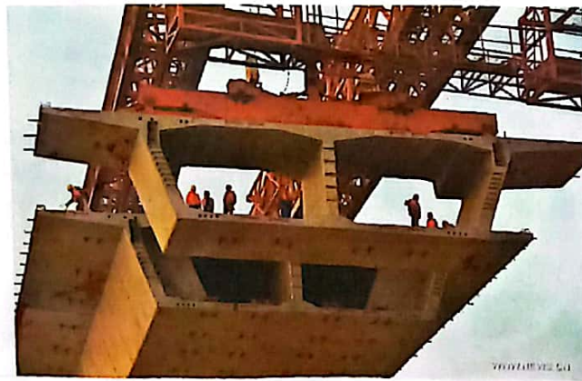
Fig : Girders of bridges.
