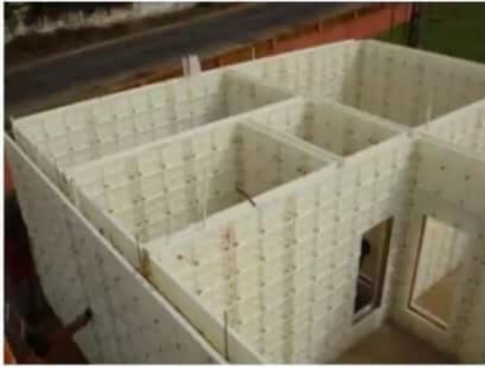
Concrete shuttering
