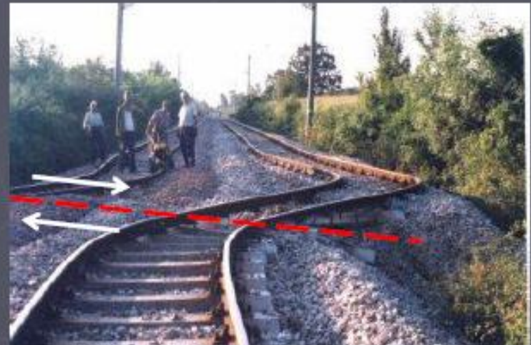
Right Lateral Slip, Izmit, Turkey, 1999 Quake
