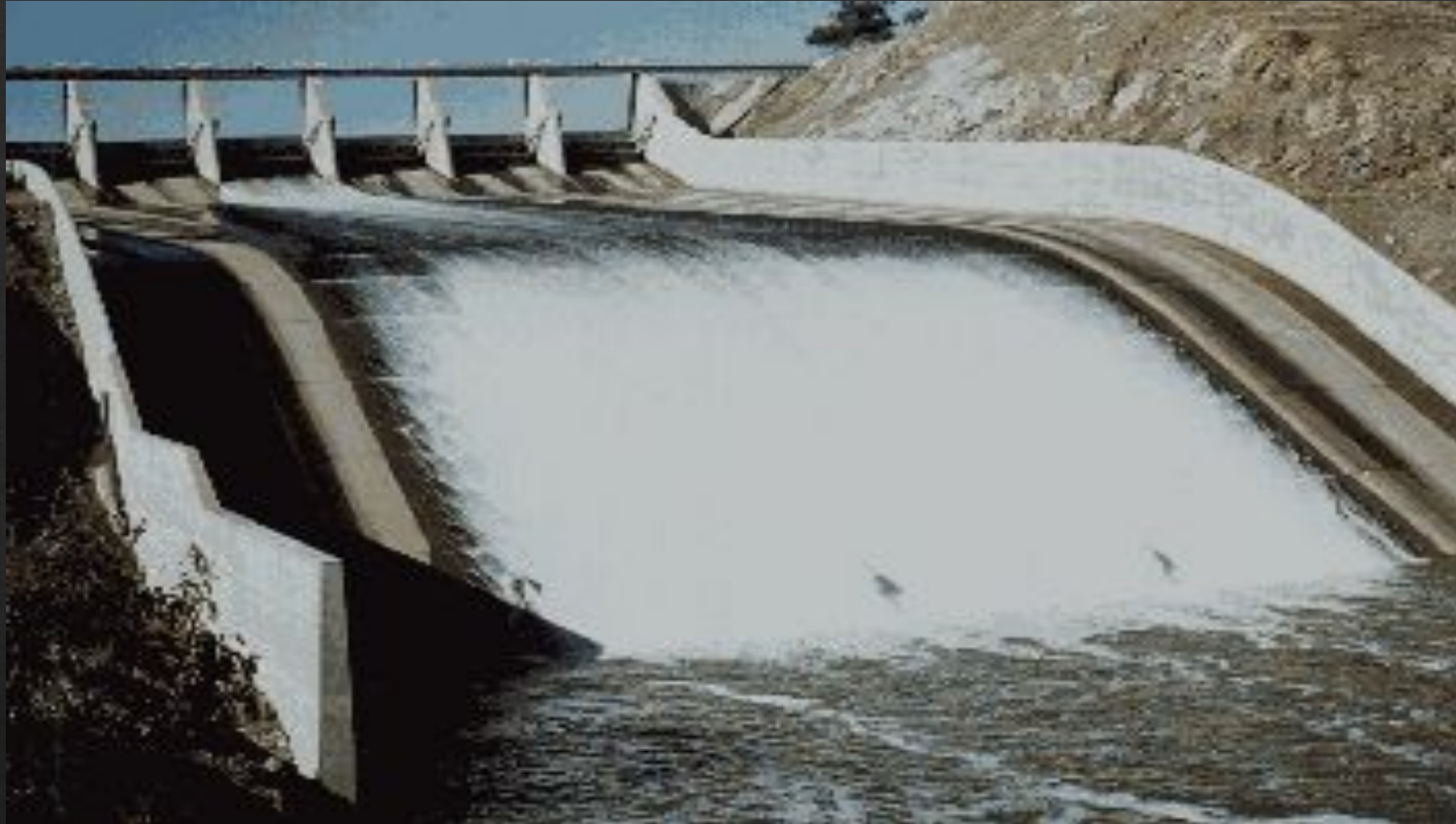
Burrendong Dam spillway showing fully lined chute and full energy dissipator.
