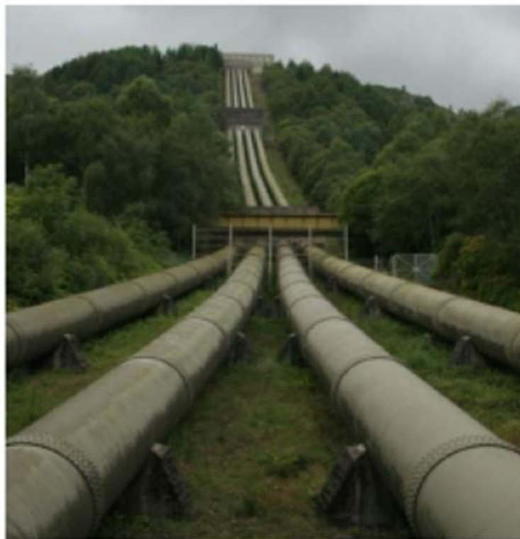
Water Transmission Systems
