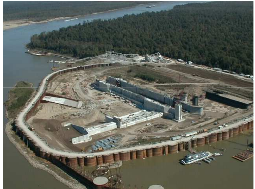
Cofferdam ( U.S. Army Corps of Engineers 2004)
