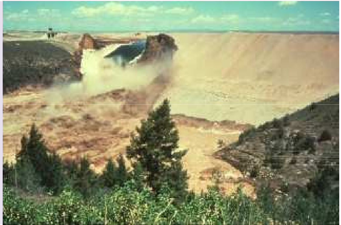
Failure of Teton Dam, June 5, 1976 (Teton River, USA)
