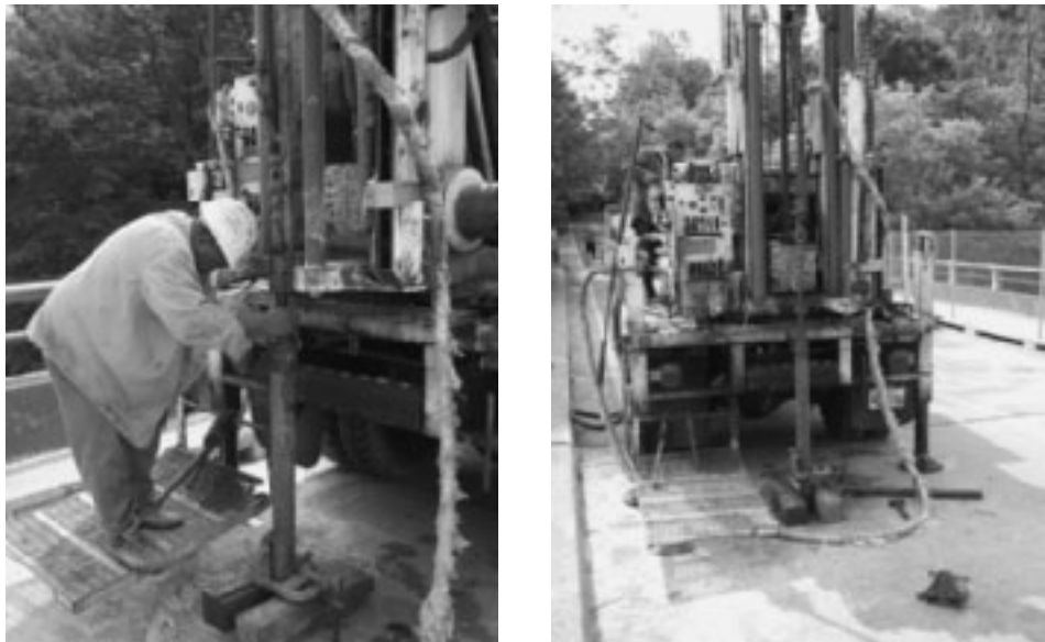
Figure 18.7 Drilling rod with split-spoon sampler lowered to the bottom of the borehole (Courtesy of Braja M. Das, Henderson, Nevada)
