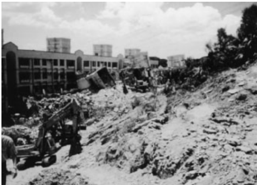
Figure 15.2 Soil and rock “fall” in a slope (Courtesy of E.C. Shin, University of Incheon, South Korea)
