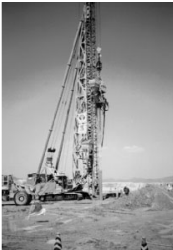
Figure 11.36 Sand drain installation in progress (Courtesy of E.C. Shin, University of Incheon, South Korea)
