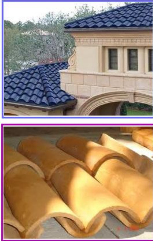
Fig. 4.3 Curved Roof Tiles
