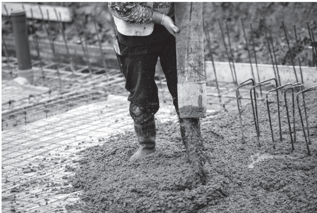
FIGURE 7.9 Placing concrete with Chute. (Fotolia/Hoda Bogdan)
