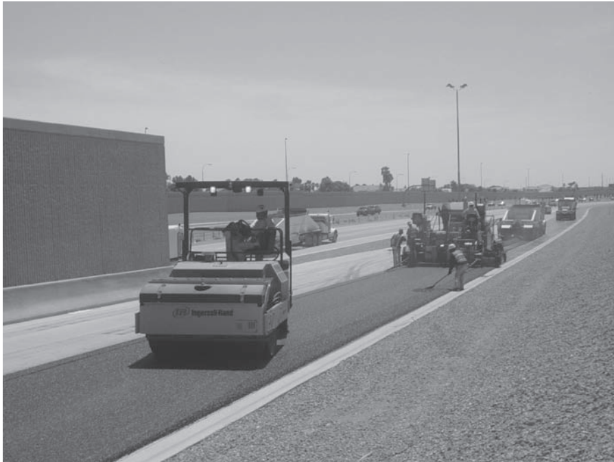
FIGURE 9.6 Compaction of asphalt concrete.
