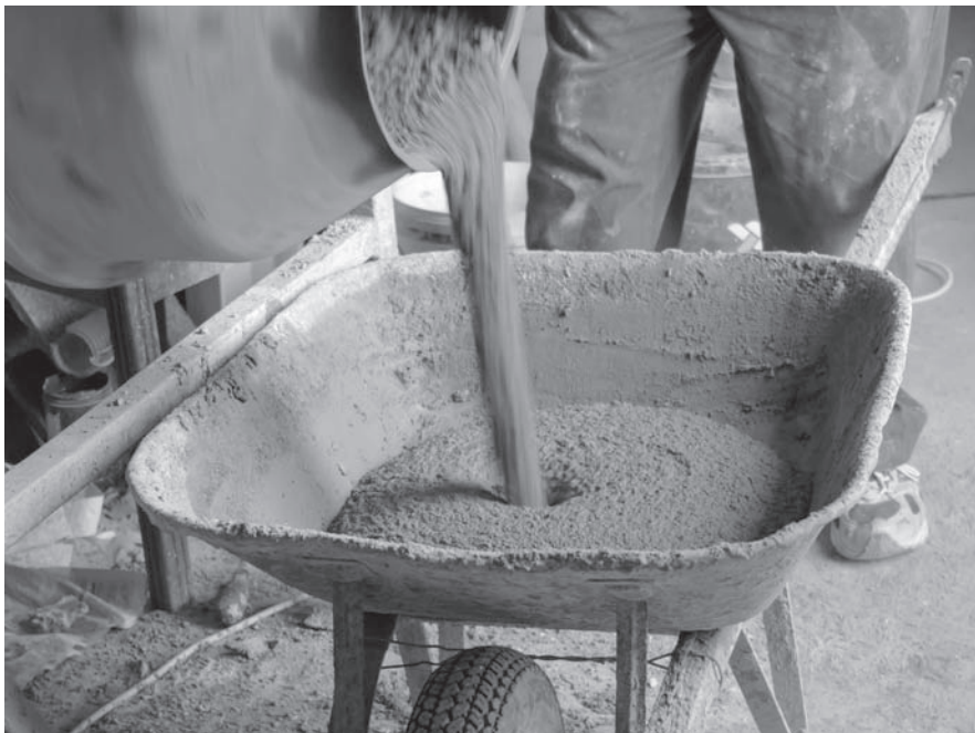
FIGURE 7.7 Loading concrete in a wheelbarrow. (Fotolia/Laure F)
