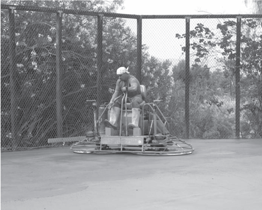
FIGURE 7.20 Finishing concrete with a power float.
