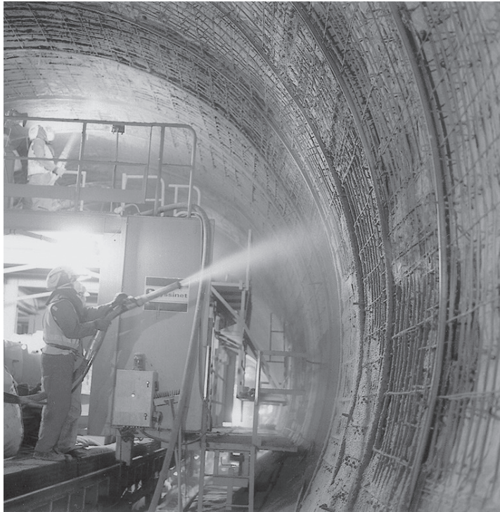
FIGURE 7.47 Shotcrete used in lining a tunnel. (Courtesy of the American Shotcrete Association)
