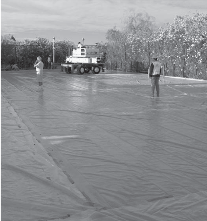
FIGURE 7.29 Curing concrete with plastic sheets.
