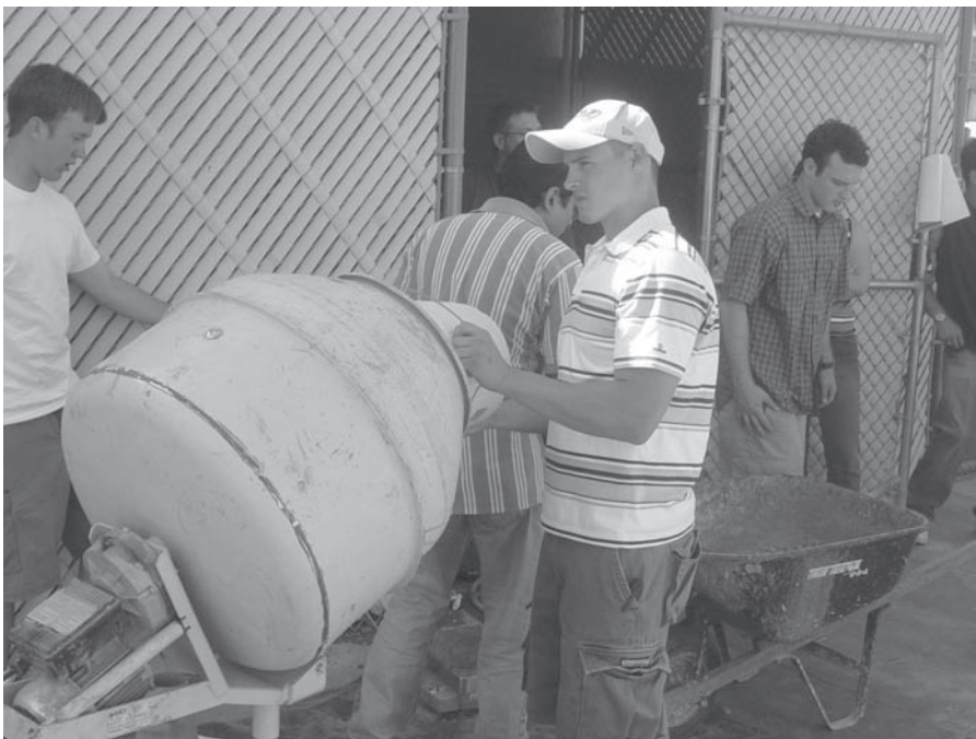
FIGURE A.30 Mixing concrete in a mixer.
