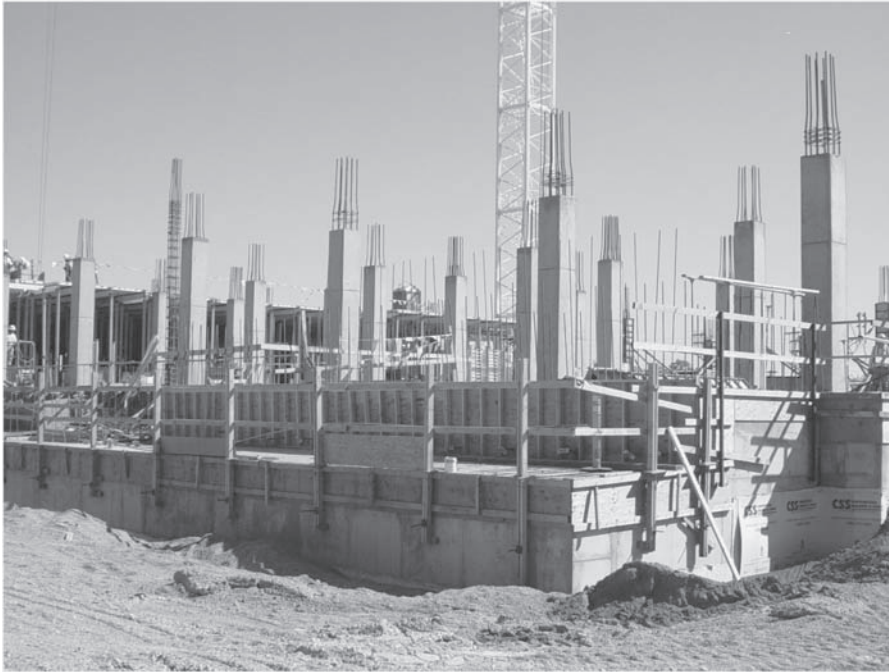
FIGURE 3.13 Steel rebars used to reinforce PCC columns.
