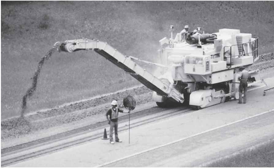
FIGURE 9.41 Milling old pavement.
