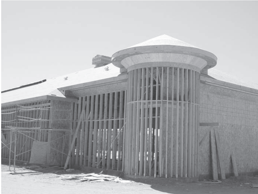
FIGURE 10.1 Wood frame used for building structural support.
