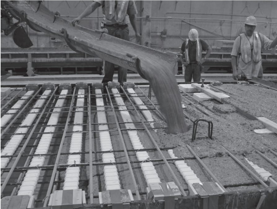
FIGURE 7.43 Placing self-consolidating concrete in a heavily reinforced slab. (Courtesy of FHWA)
