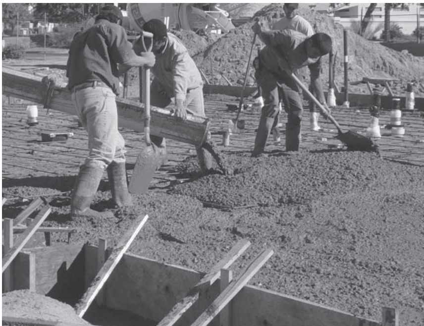
FIGURE 7.8 Placing concrete slab.
