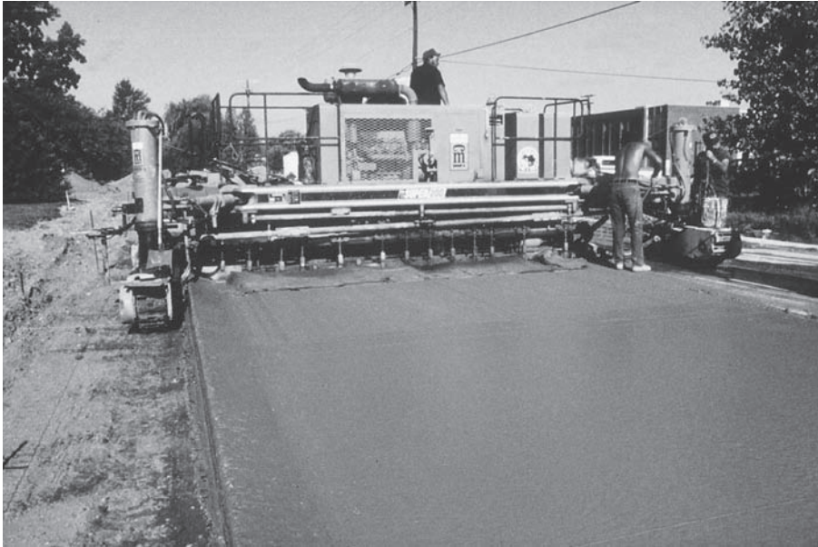
FIGURE 7.10 Placing concrete pavement with a slip-form paver.
