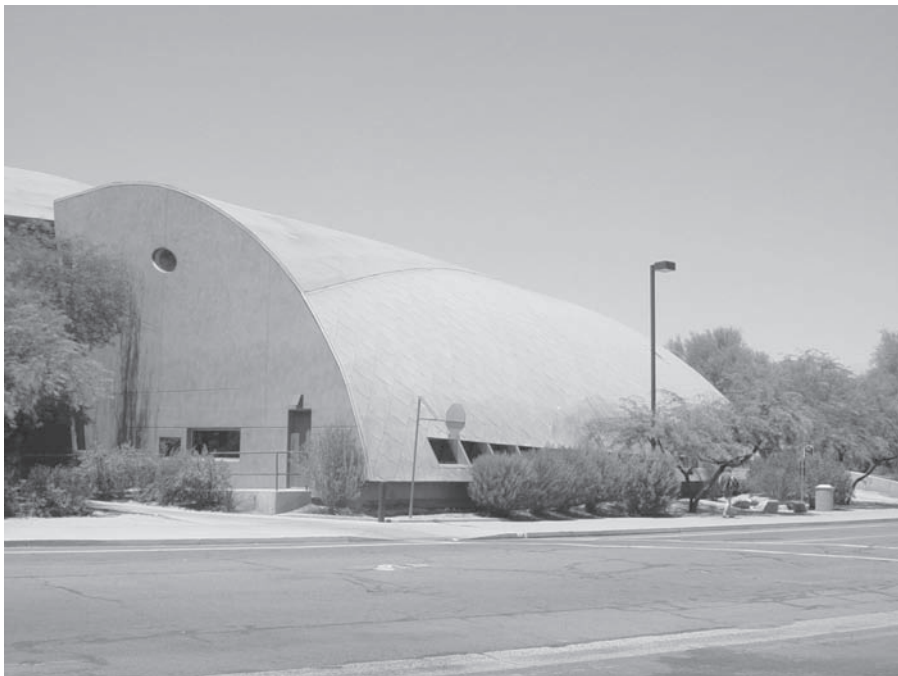
FIGURE 4.2 Building facade made of aluminum.
