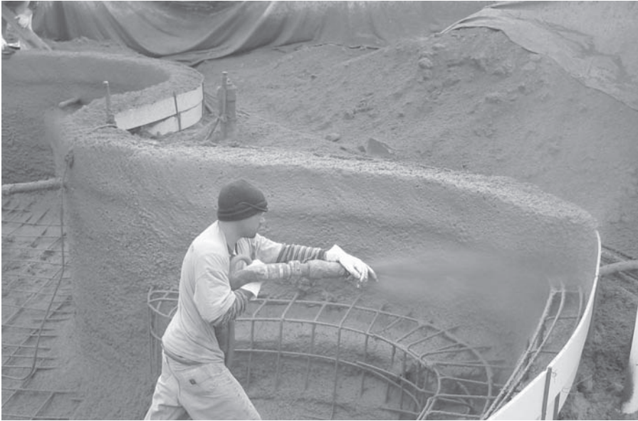
FIGURE 7.46 Constructing a swimming pool using shotcrete. (Courtesy of the American Shotcrete Association)
