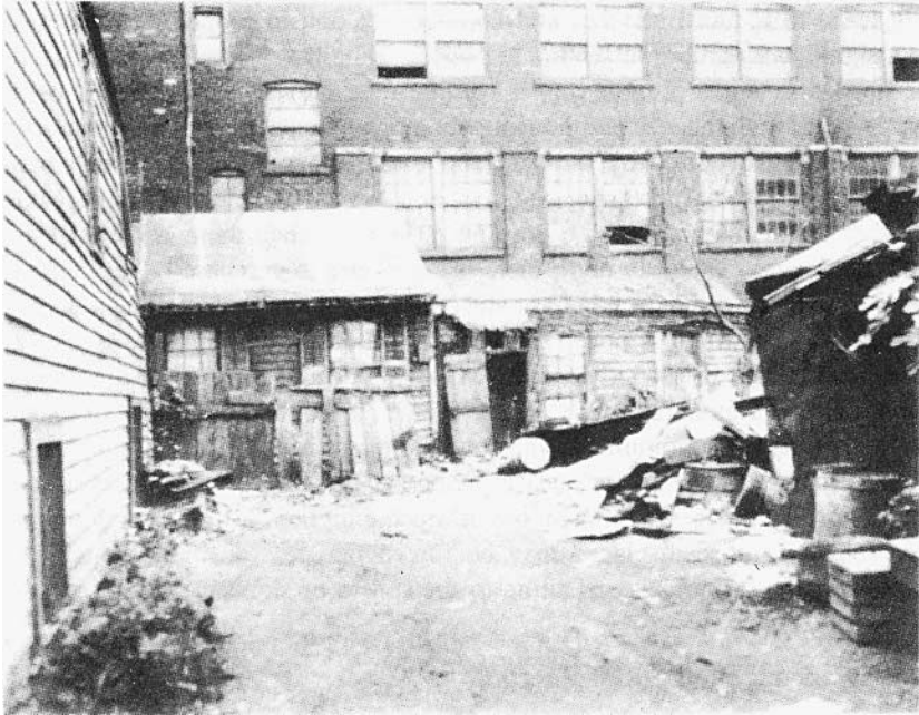
Figure 10-2 Run-down, filthy, vermin-infested backyards present many real health hazards.
