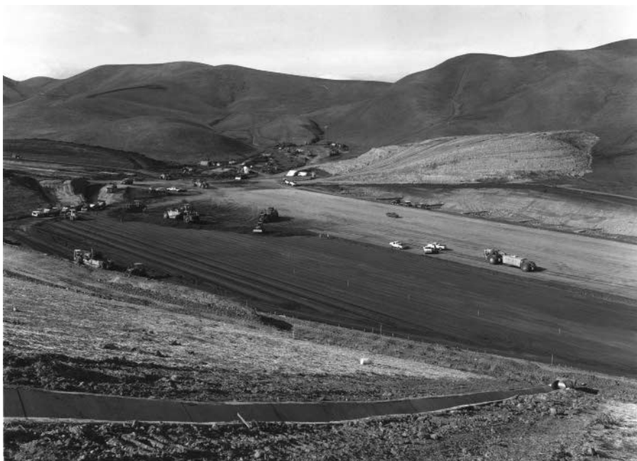
Figure 5-25 Development of large ravine landfill site. Equipment is compacting sub-base of landfill in preparation for placement of geomembrane liner.
