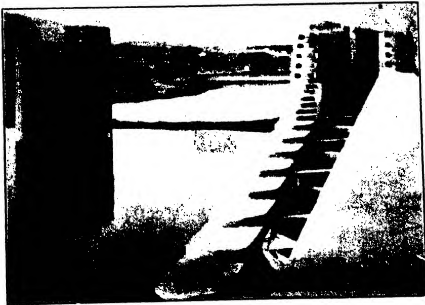
A view of the fish ladder along the right divide wall Trimmu Weir. Fig. 10 (b).
