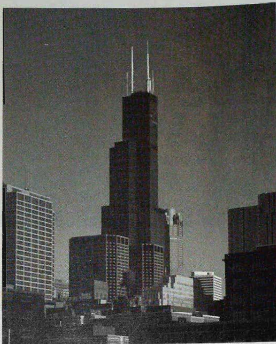
1730 ft Sears Tower, Chicago (photo courtesy of Galen R. Frysinger)
