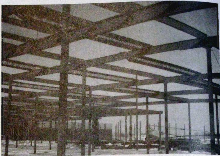
Beams, including open-web joists, channels, and W (wide-flange) shapes, along with tubular columns. (Photo by C.G. Salmon)
