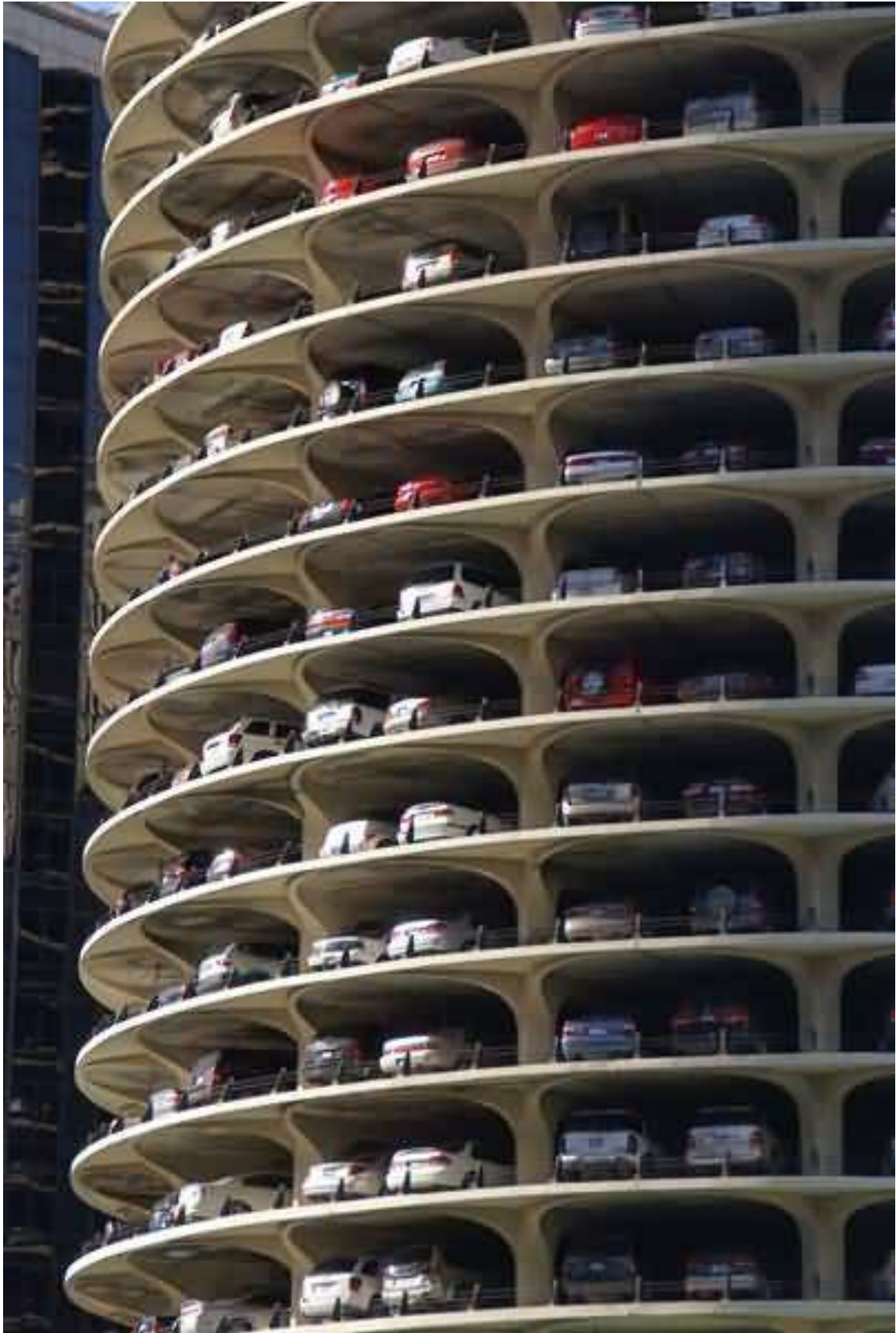
Multi-storied off street parkings
