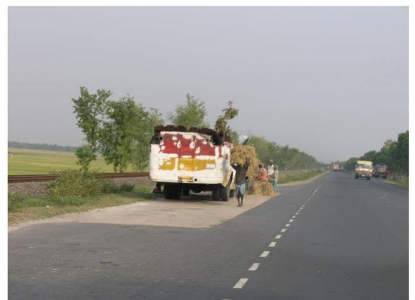
Use of Rigid Pavement at Waiting Area
