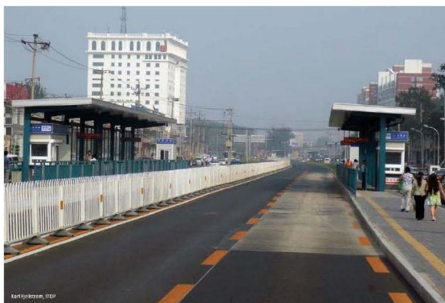
Use of Rigid Pavement at Bus Stoppage
