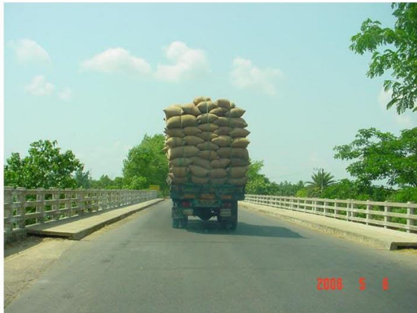
Controlling Overloading Problems
