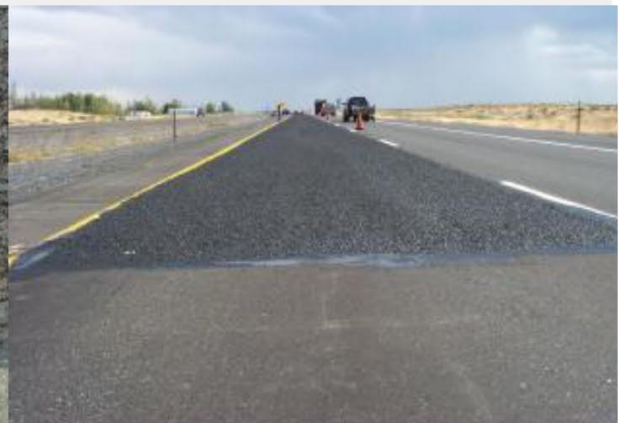
Figure 4: Finished micro-surface.
