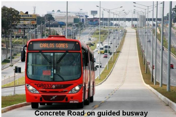
Concrete Road on tight r.o.w. (Roller inaccessible)
