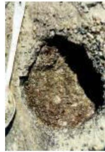
Stripping at bottom of hole
