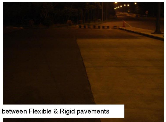
Higher watt bulbs needed for asphalt pavement
