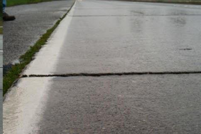
Figure 2: Faulting close-up.
