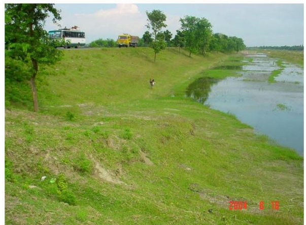
Maintaining Embankment Stability
