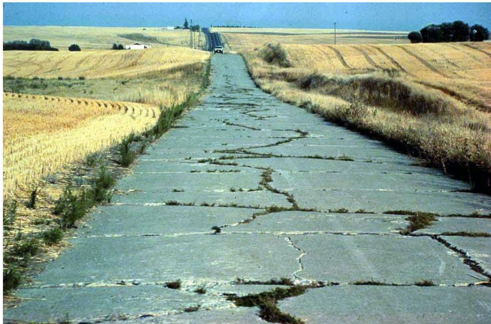
An older Portland Cement Concrete road (USA, paved in 1919)
