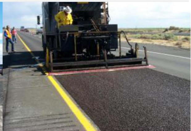
Figure 2: Micro-surfacing placement.
