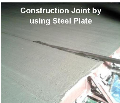
Construction Joint by using Special Planner
