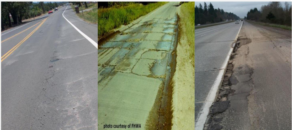
Figure 1: Pumping in action.
