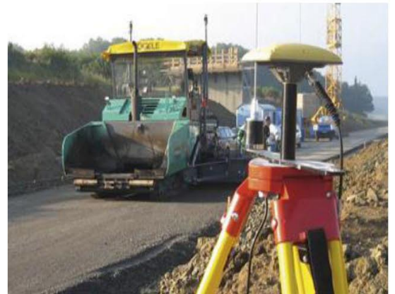
Paver with GPS (3D Positioning) System
