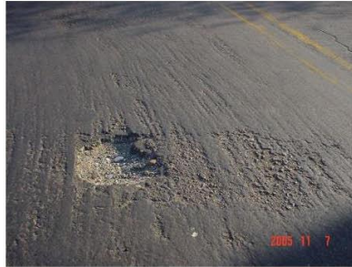
Developing pothole
