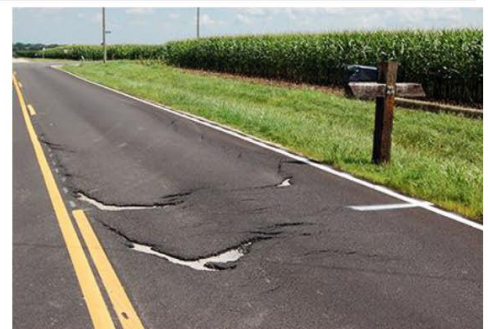
Slippage cracking
