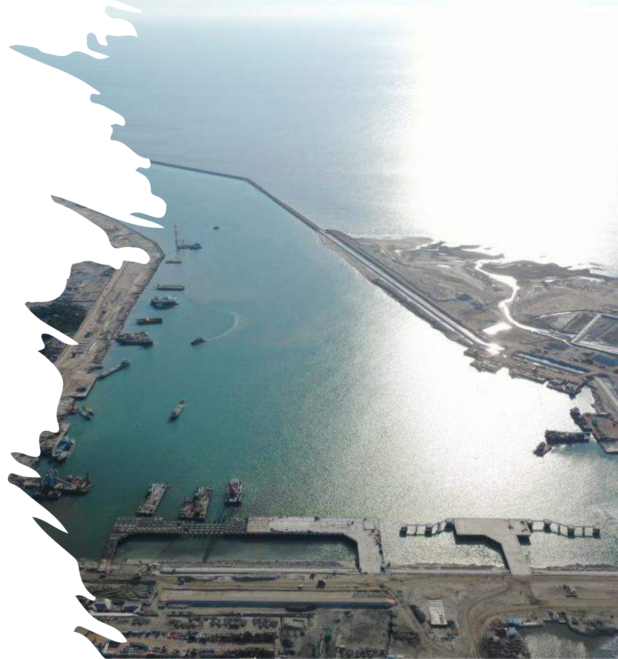
tarbari 2x600 MW USC Coal Fired Power Plant Project
